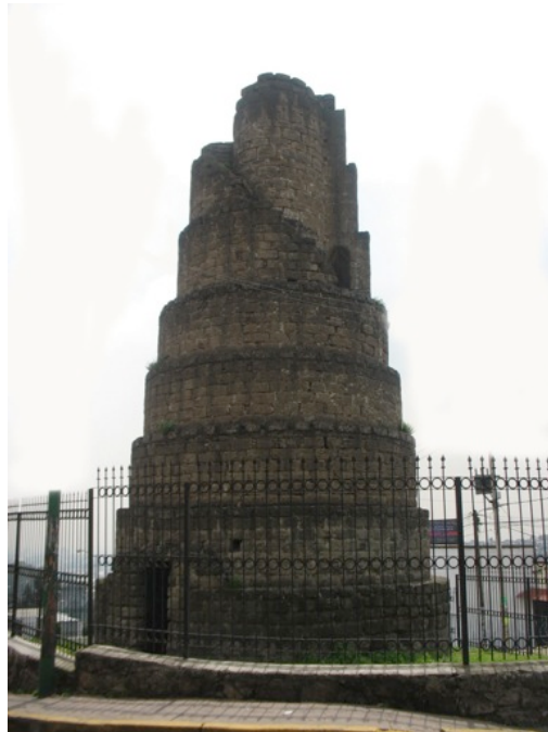
Figure 3. 4: Unknown Author. Caracol , eighteenth century structure, part of the hydraulic system to bring water to the shrine of Our Lady of Remedios. Picture by author
