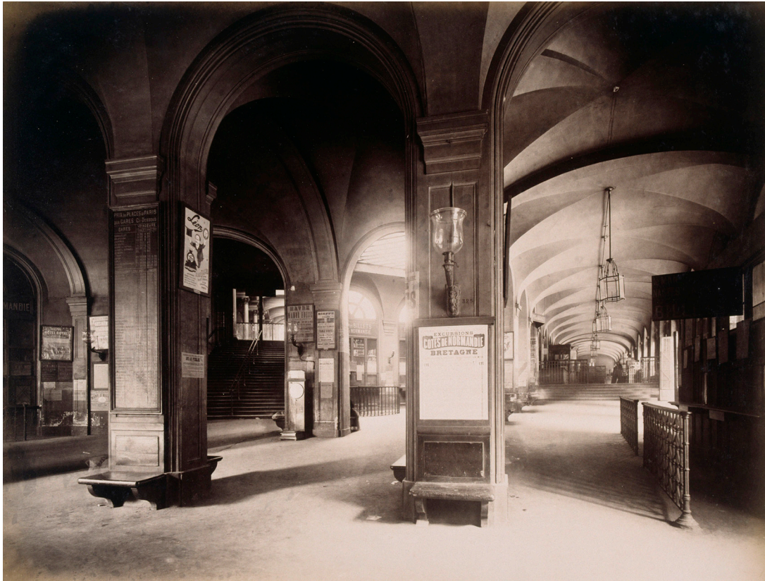
2.26. Durandelle, Gare Saint-Lazare: Normandie departures, baggage hall, stairs to waiting rooms, 1887. Albumen print. Collection Musée d'Orsay PHO 2000 9 7. Image courtesy RMN.
