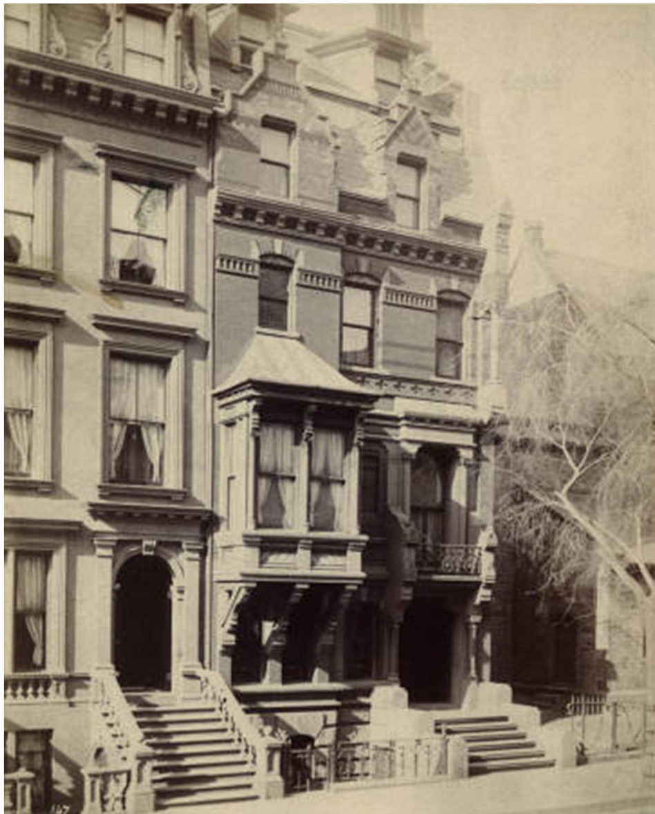
2.39. Unknown photographer, possibly Albert Lévy, Ware and Van Brunt, Residence 38th St. near Madison Ave, New York NY, c. 1883. Photograph. In Albert Lévy's Architectural Photographic Series 1, no. 147. Art Institute of Chicago Architecture Photograph Collection RBA Digital File name 59270.
