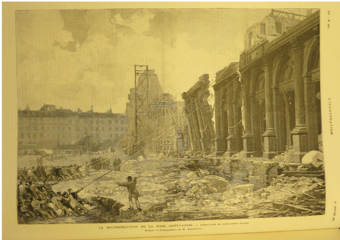
2.27. Reconstruction of the gare Saint-Lazare. Demolition of the old façade. After M. Durandelle's photograph. Engraving. In L'Illustration 91, no. 2344 (28 January 1888): 56. Collection Canadian Centre for Architecture, Montréal PER W.I446.
