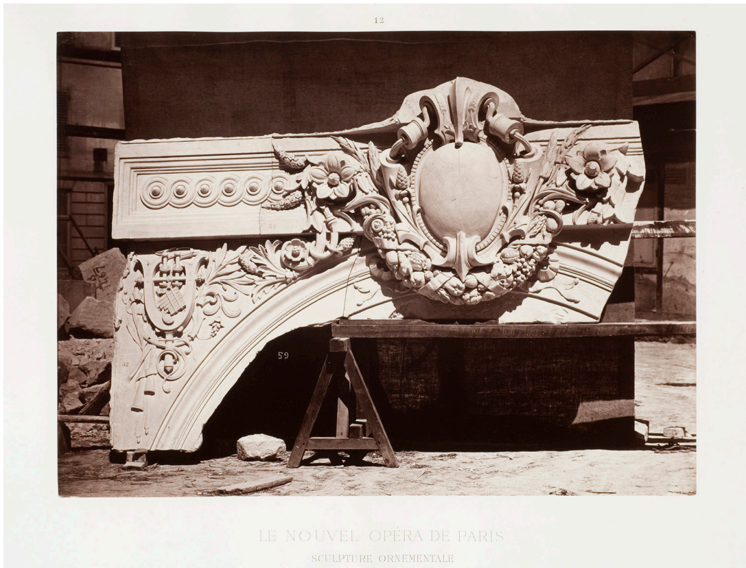
1.19. Louis-Émile Durandelle, View of a keystone and tympanum of the lower part of the Ticket Lobby, c. 1868. Albumen silver print. In Charles Garnier, Le Nouvel Opéra de Paris, Sculpture ornementale (Paris: Ducher et Cie., 1876), plate 12. Collection Centre Canadien d'Architecture/Canadian Centre for Architecture, Montréal PH1979:0162.04:012.
