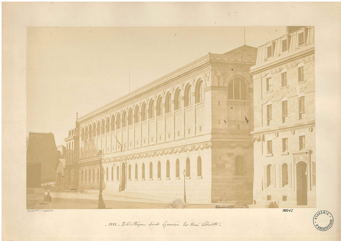
2.54. Louis-Auguste et Auguste-Rosalie Bisson (Frères), Façade of the Bibliothèque Sainte-Geneviève in 1852. Salted paper print probably coated with albumen, on mount. Académie d'Architecture 492.
