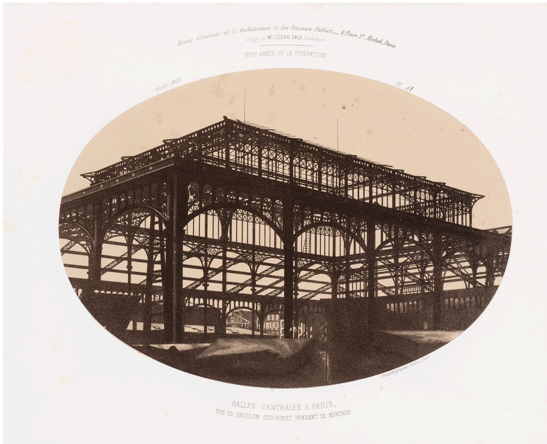
5.3. Halles Centrales, Paris: View of the southwest pavilion under construction, 1856. Photograph. In Revue générale de l'architecture et des travaux publics 14 (1856): plate 41. Collection Centre Canadien d'architecture/Canadian Centre for Architecture, Montréal PER W.R484.
