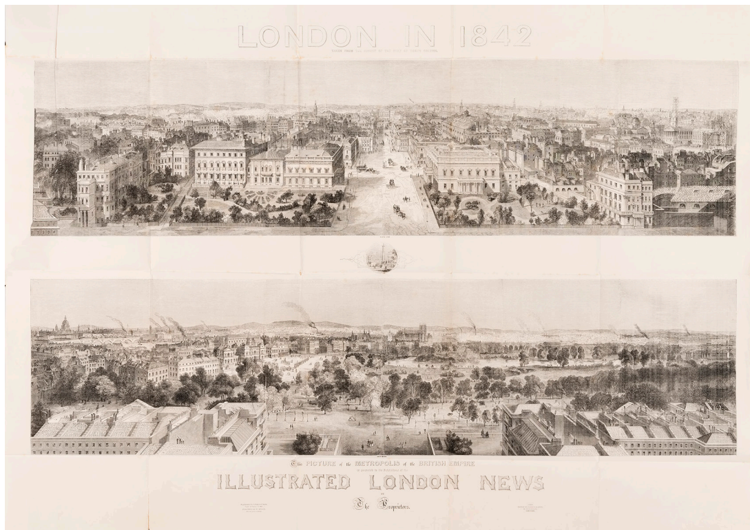
2.10. London in 1842, Taken from the summit of the Duke of York's column [The "Colosseum Print"], 1843. Engraving. In Illustrated London News 2, no. 36 (8 January 1843). Collection Centre Canadien d'Architecture / Canadian Centre for Architecture, Montréal PER W.I444.
