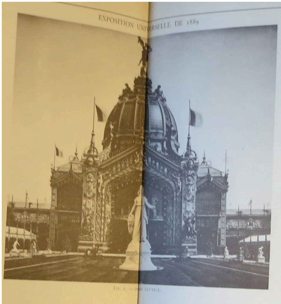
3.15. Exposition Universelle of 1889. Dôme Central. Glyptographie. In Nouvelles Annales de la Construction 35, no. 416 (1889): plates. 36–37, fig. 1. Collection Centre Canadien d'Architecture/Canadian Centre for Architecture, Montréal PER W.N68. Photograph by Peter Sealy.
