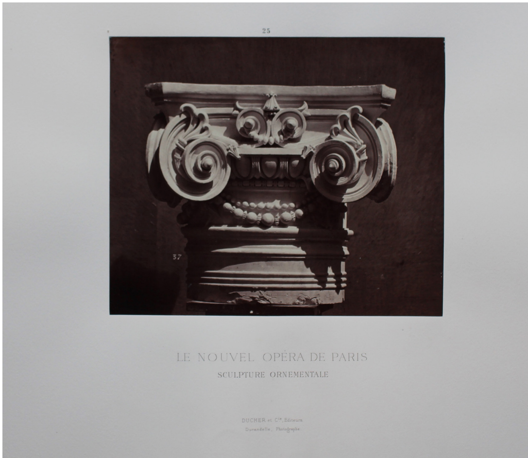
1.20. Louis-Émile Durandelle, Column capital from the Circular Vestibule, 1875 or earlier. Albumen silver print. In Charles Garnier, Le Nouvel Opéra de Paris, Sculpture ornementale (Paris: Ducher et Cie., 1876), plate 25. Collection Centre Canadien d'Architecture/Canadian Centre for Architecture, Montréal PH1979:0162.04:037. Photo-graph by Peter Sealy.
