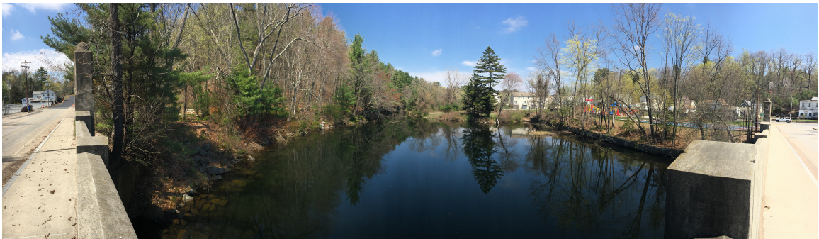
Figure 10. Area surrounding the Swift River in the developed sample site. This panorama looking north of the developed sample site shows development within the 25-foot riverfront area along the eastern edge of the Swift River. The western edge is bordered by a large wall (possible levee), trail, and small section of temperate seasonal forest. (photo by author, 2017).
