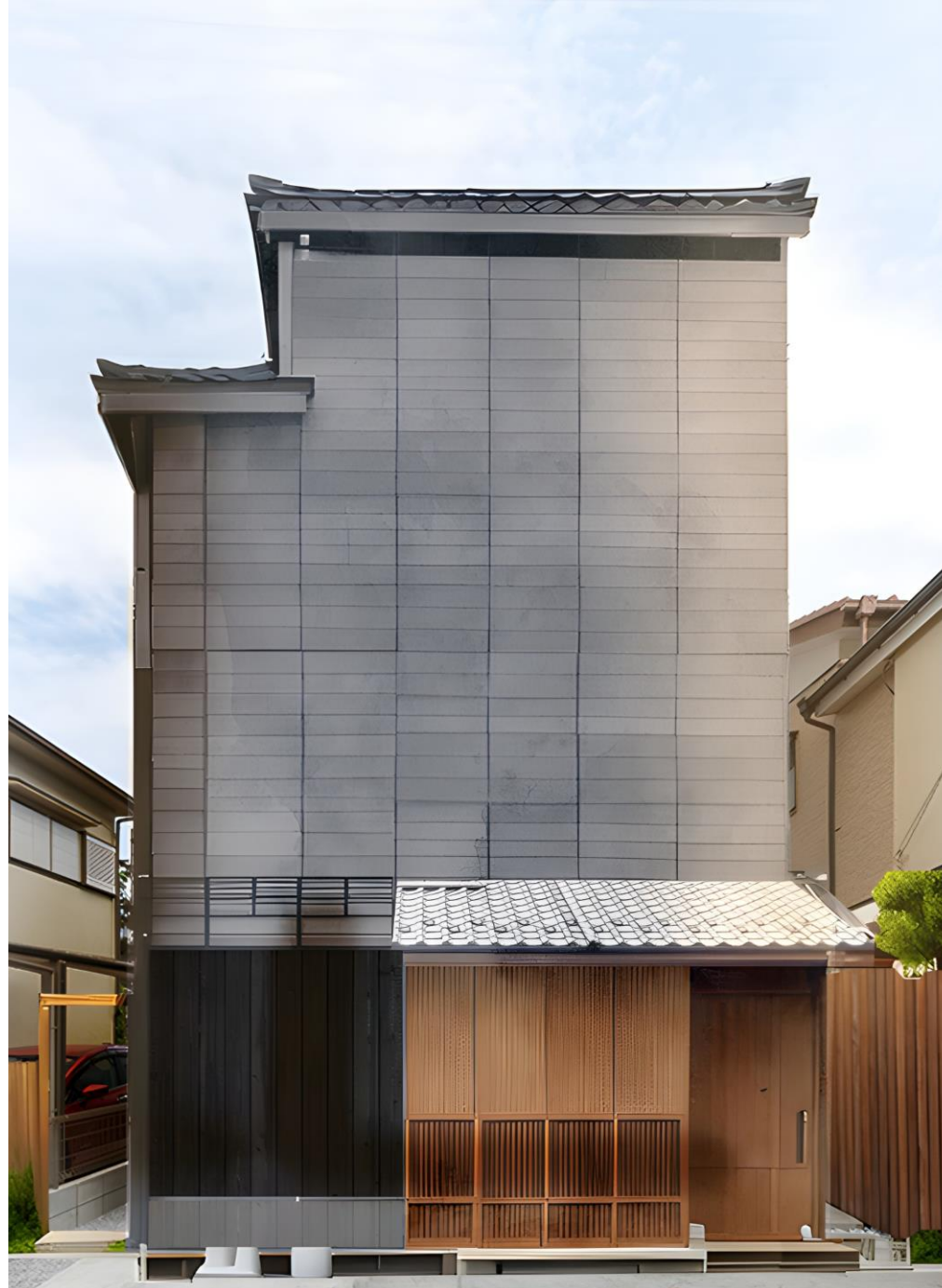
Transformed façade propose materiality palette mixed from the selected eras. Sugi-ban and wooden louver doors, ceramic tiles.
