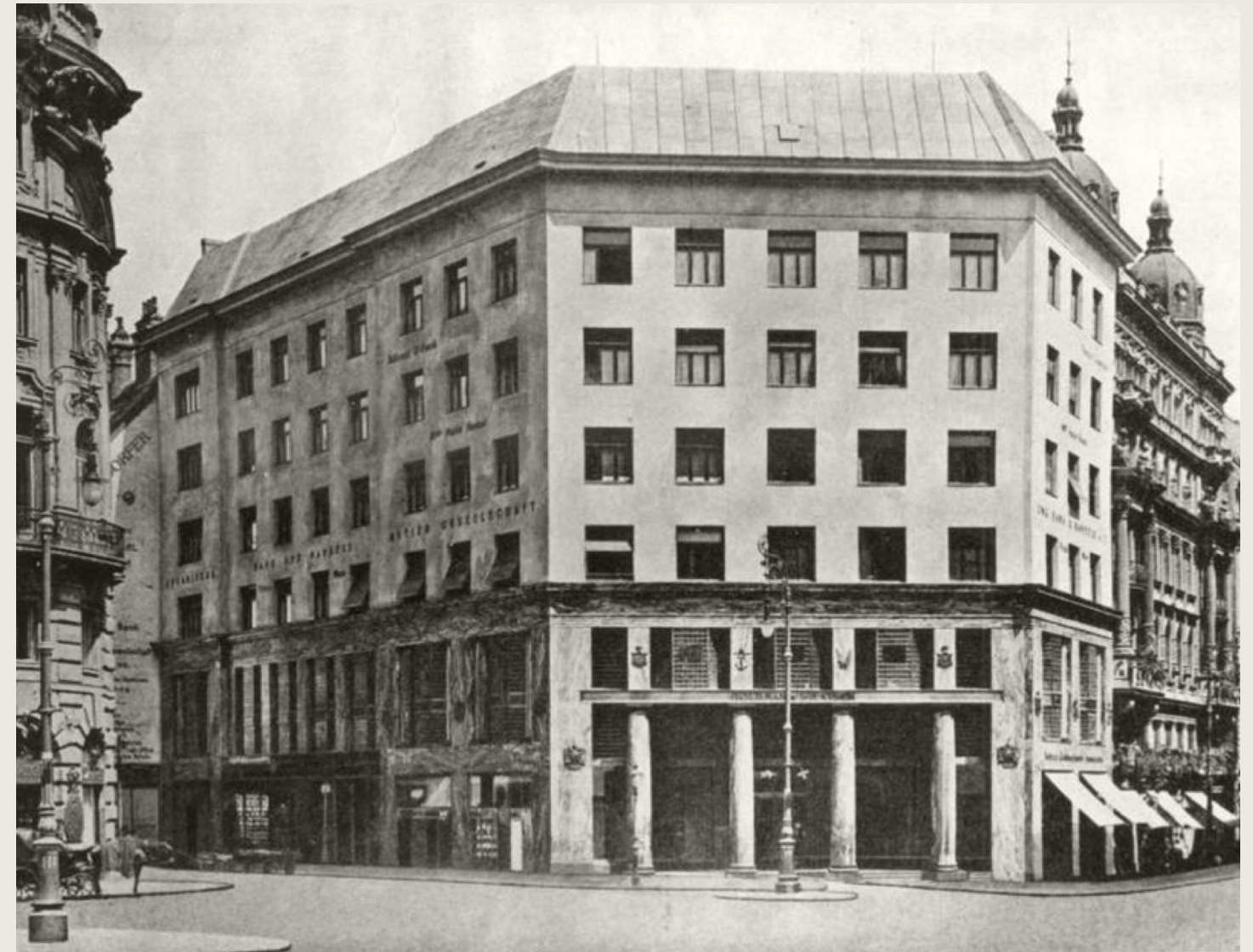
Adolf Loos, Looshaus, Vienna, Austria, 1911
