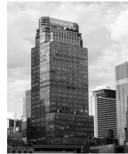
F [ McGraw Hill Building ] Location 330 West 42nd Street New York, NY Year 1930 (2023) Program: Office > Residential
