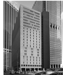
G [ 25 Water Street ] Location 4 New York Plaza, New York, NY 10004 Year 1969 (planned) Program: Office > Residential
