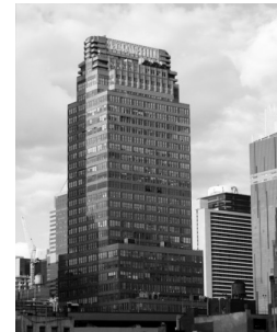
F [ McGraw Hill Building ] Location 330 West 42nd Street New York, NY Year 1930 (2023) Program: Office > Residential
