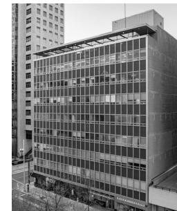
P [ Taylor Building ] Location 805 8th Ave SW, Calgary, AB T2P 1H7, Canada Year 1958 (planned) Program: Office > Residential
