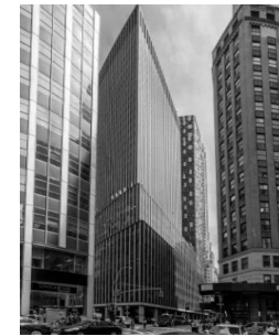
H [ 55 Broad Street ] Location 55 Broad St, New York, NY 10004 Year 1967 (planned) Program: Office > Residential
