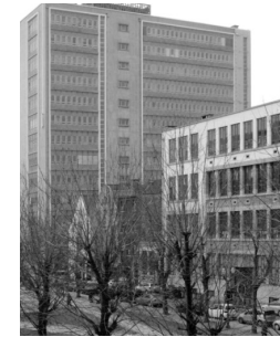
J [ The Cosmopolitan ] Location Quai aux Pierres de Taille 16/281000 Bruxelles, Belgium Year 1960 (2019) Program: Office > Residential
