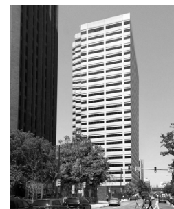
O [ Franklin Tower ] Location 200 N 16th St, Philadelphia, PA 19102 Year 1975 (2017) Program: Office > Residential
