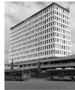
I [ Terminus House ] Location Terminus St, Harlow, CM20 1XA, United Kingdom Year 1975 (2018) Program: Office > Residential
