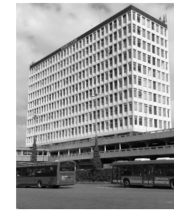
I [ Terminus House ] Location Terminus St, Harlow, CM20 1XA, United Kingdom Year 1975 (2018) Program: Office > Residential
