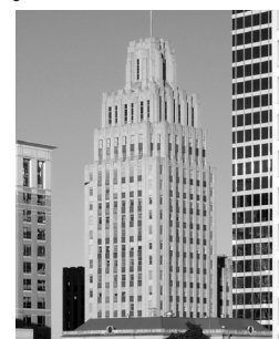
B [ The Reynolds Building ] Location 51 E. 4th St., Winston-Salem, North Carolina Year 1929 (2016) Program: Office > Residential
