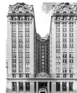
A [ 49 Chambers ] Location 51 Chambers St., Manhattan, New York Year 1912 (2017) Program: Office > Residential
