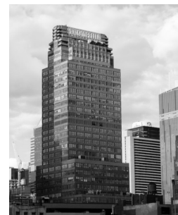
F [ McGraw Hill Building ] Location 330 West 42nd Street New York, NY Year 1930 (2023) Program: Office > Residential
