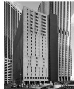
G [ 25 Water Street ] Location 4 New York Plaza, New York, NY 10004 Year 1969 (planned) Program: Office > Residential
