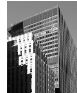
E [ 160 Water St ] Location 160 water street New York, NY 10038 Year 1972 (2023) Program: Office > Residential
