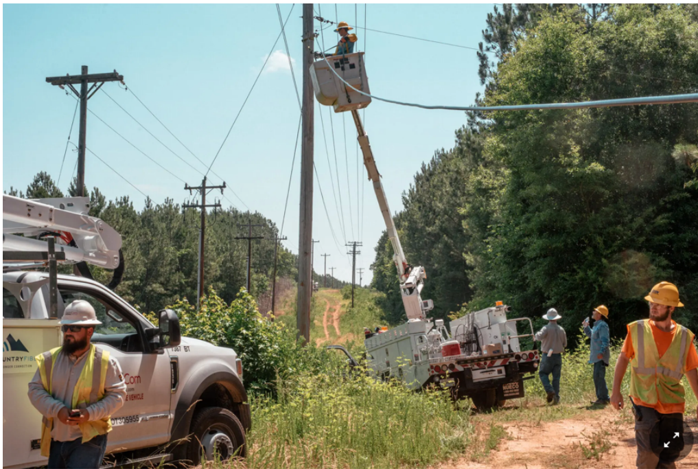
Figure 1. Fiber-optic installation.
