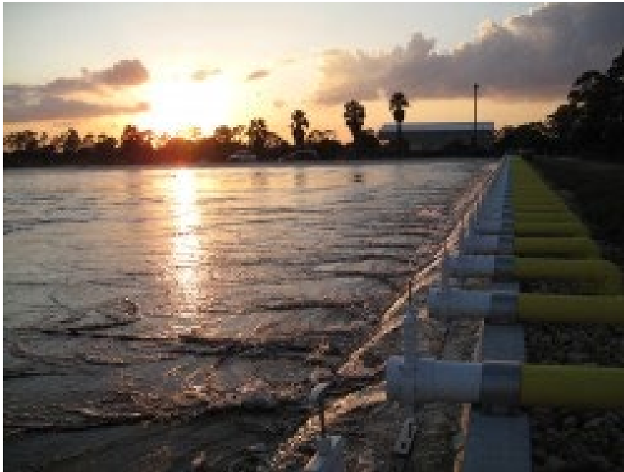
Figure 6. ATS inflow pipes.
