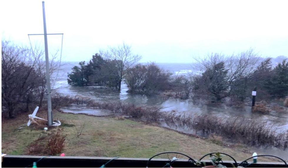
Figure 26. Storm surge on Old Mill Blvd.
