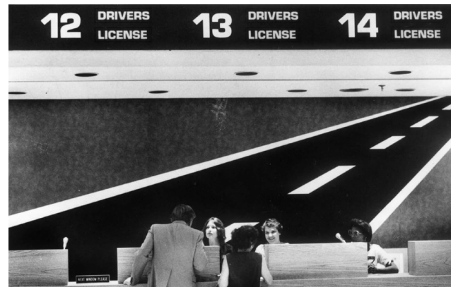
1983. drivers get lisences at DMV office in Richmond, VA. Richmond Times-Dispatch, "From the Archives: The Virginia Department of Motor Vehicles." Jan. 31, 2018. Staff photo.
