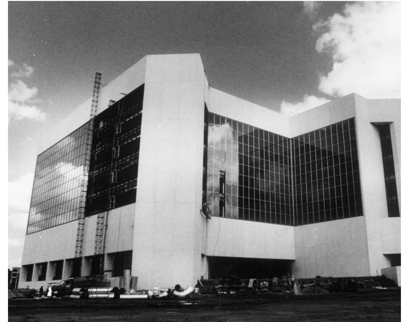
1979. The New Headquarters of the Divison of Motor Vehicles has taken on a glassy look now that many of the windows have been installed. the $13M building is scheduled to be completed in early 1979 according to DMV. Richmond Times-Dispatch, "From the Archives: The Virginia Department of Motor Vehicles." Jan. 31, 2018. Staff photo.
