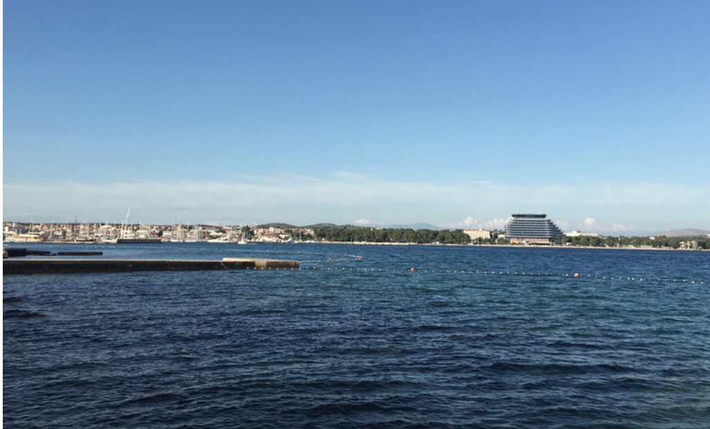
Fig. 3 Hotel Olympia Sky, Vodice. 2015-2017. Architects: Vulin i Ileković. Photo: by the author, 2018.
