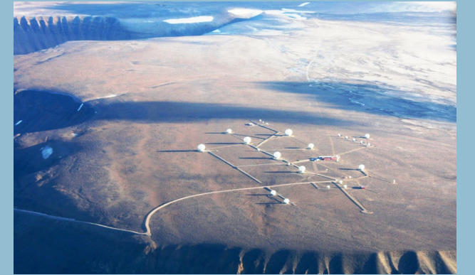
FIG. 30 Svalbard Satellite Station. Norway.
