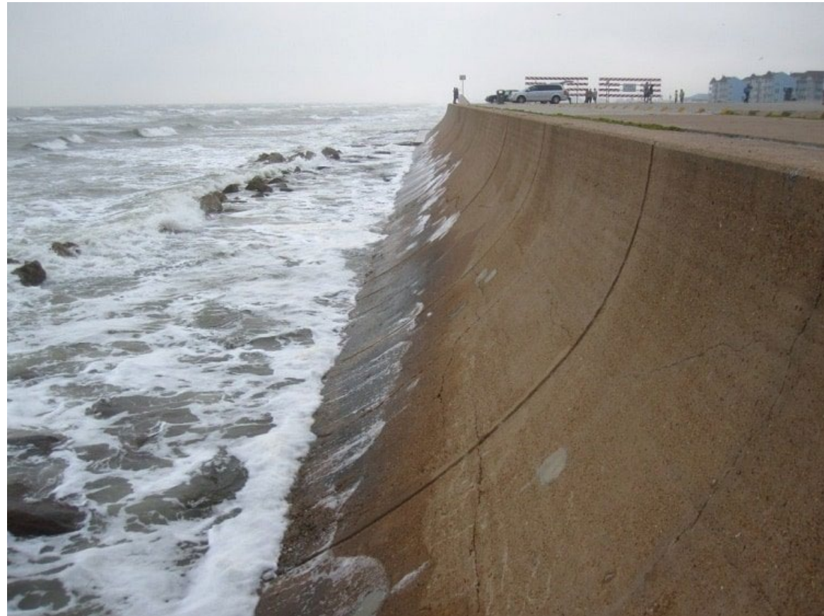
FIG. 51 Curved Concrete Coastal Infrastructure
