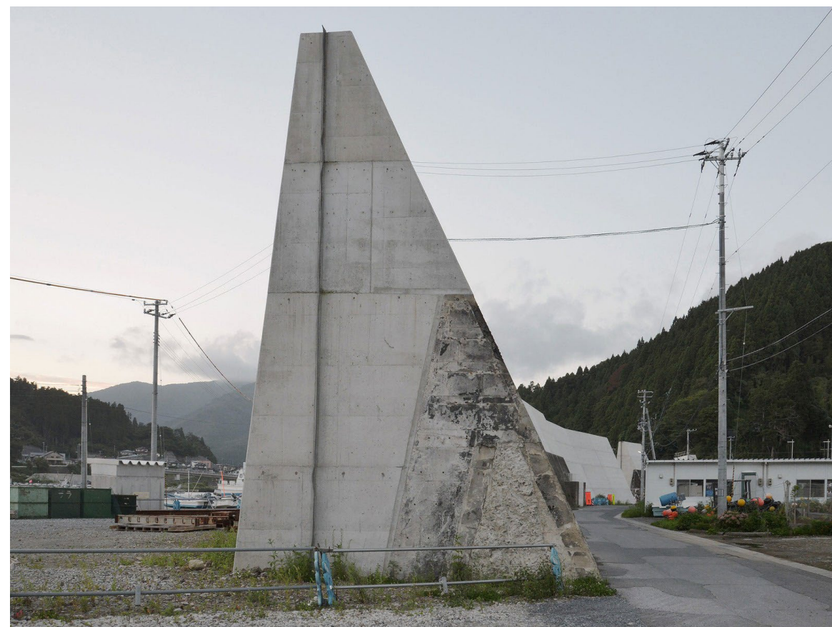
FIG. 53 Seawall. Ryori Bay, Iwate prefecture, Japan.
