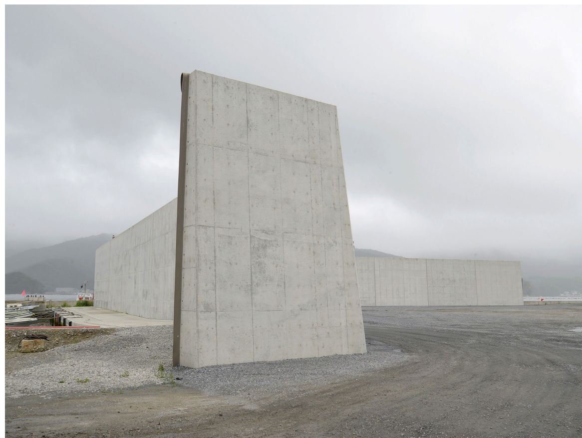
FIG. 52 Seawall. Ofunato Bay, Iwate prefecture, Japan.
