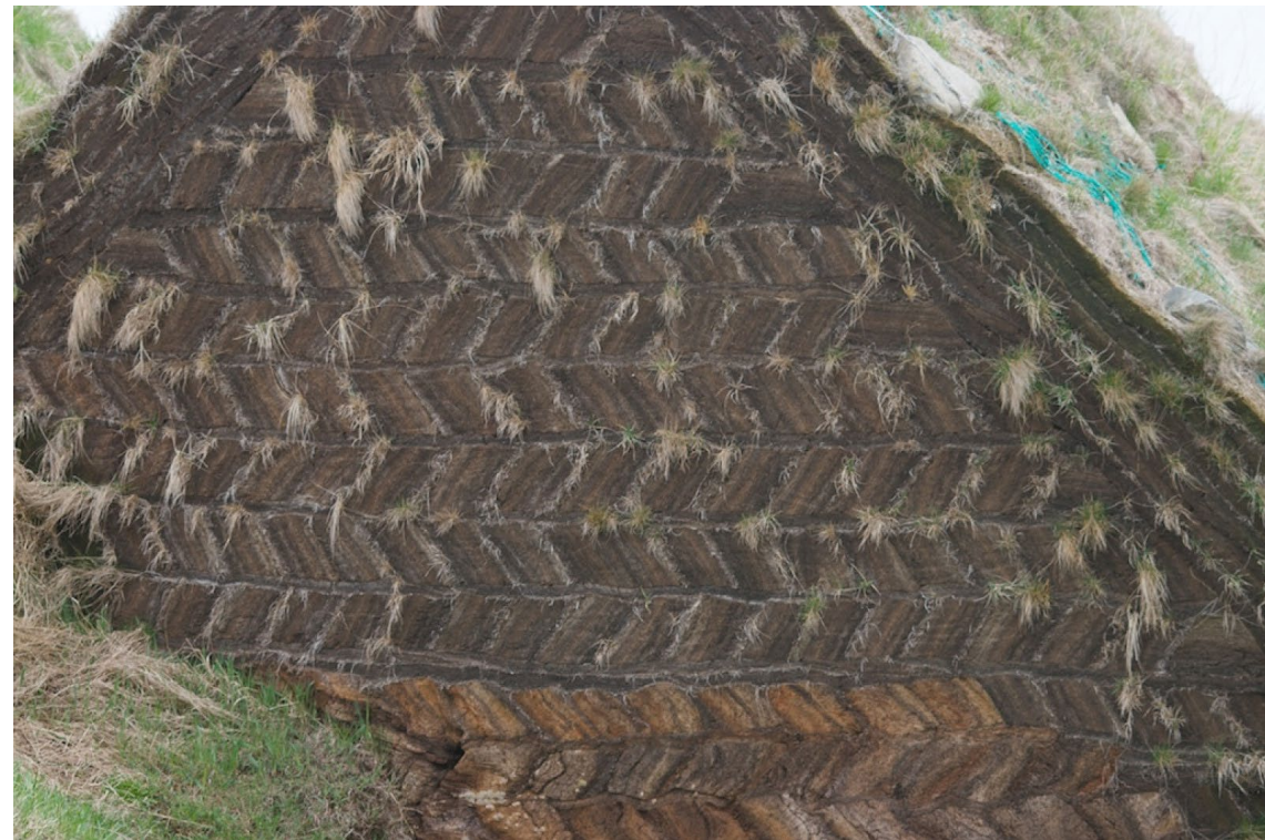
FIG. 39 Turf arranged into herringbone pattern.
