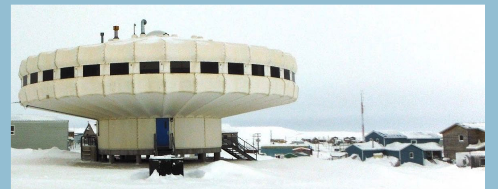
FIG. 29 Igloolik Research Station. Canada.
