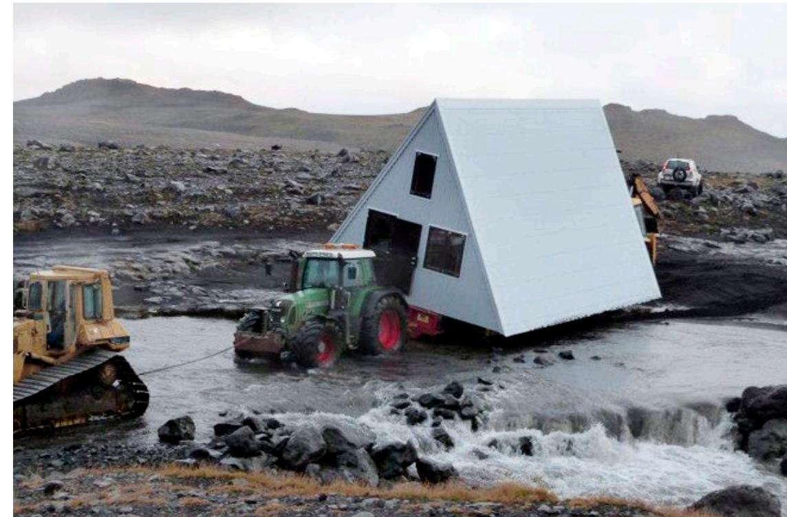
FIG. 41 Building in Fragile Nature.
