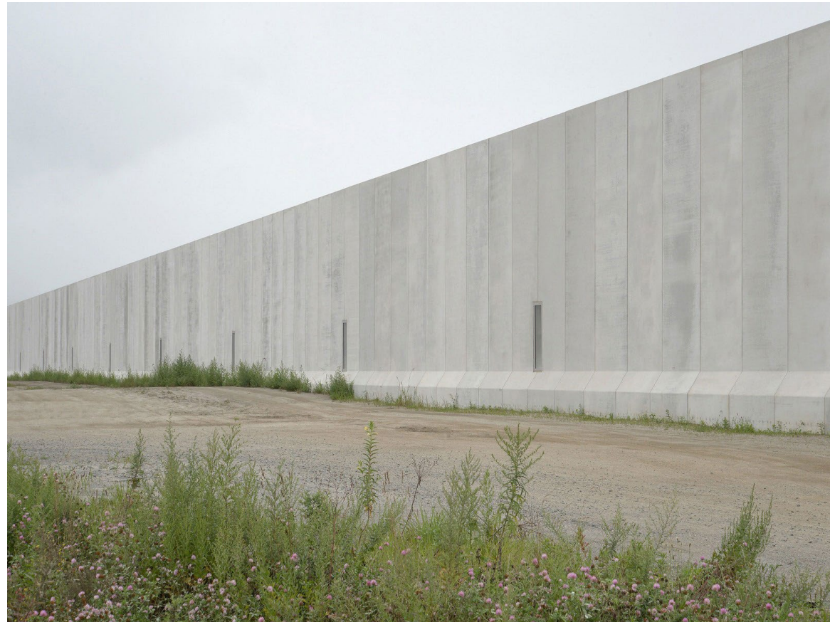
FIG. 54 Seawall. Miyako Bay, Iwate prefecture, Japan.
