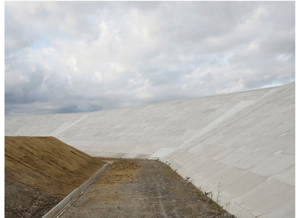
FIG. 55 Seawall. Kesenuma Bay, Miyagi prefecture, Japan.
