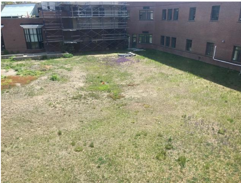
Figure 20 Second story classroom view of CMS courtyard. Annmarie Barone, Spring 2021
