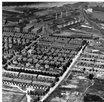
Roebing Steel Mill
