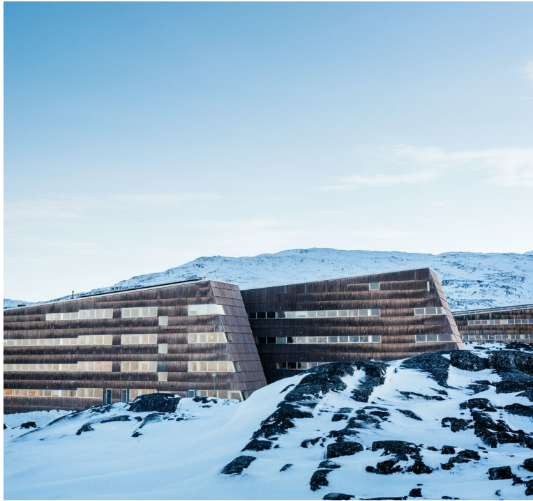
The University of Greenland occupies a collection of buildings with “uncolored” wooden facades.
