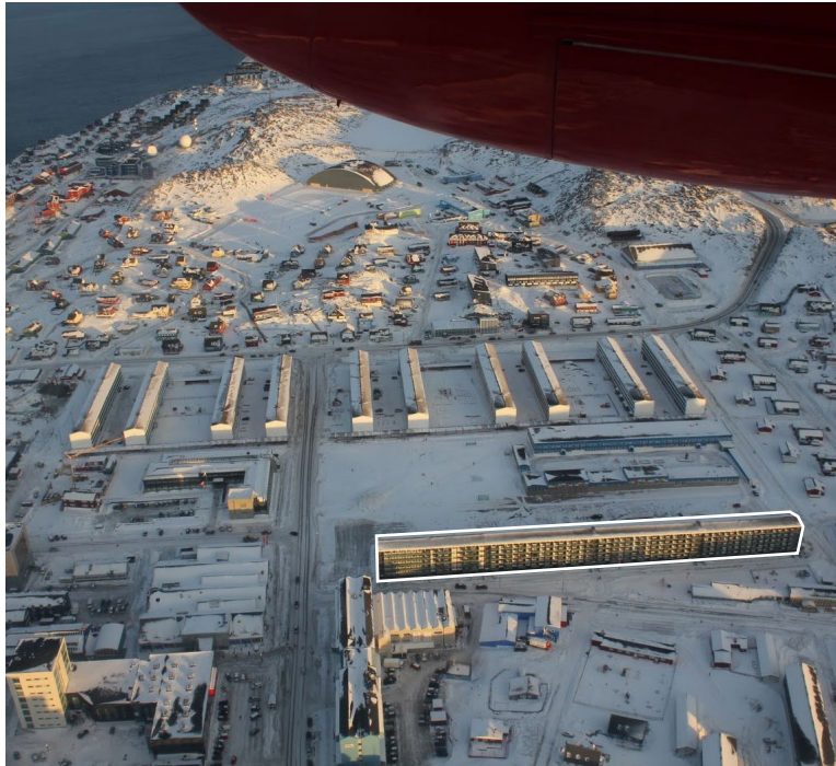
Highlighted in white is Nuuk's infamous Block P—a 200m-long, five-storey high building that testified to the failure of Danish housing policy in the 1960s.
