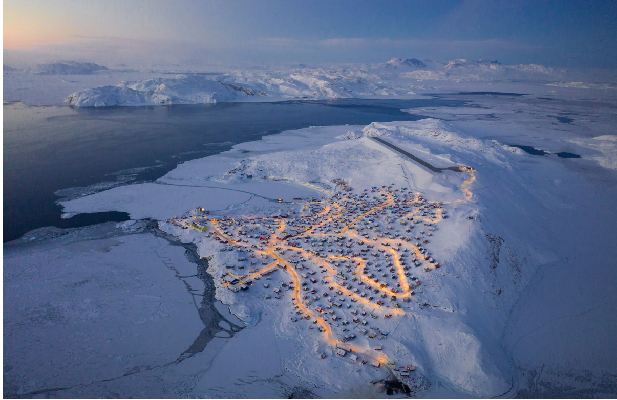
Airport as crucial infrastructure connected to the small village of Upernavik, northwestern Greenland.
