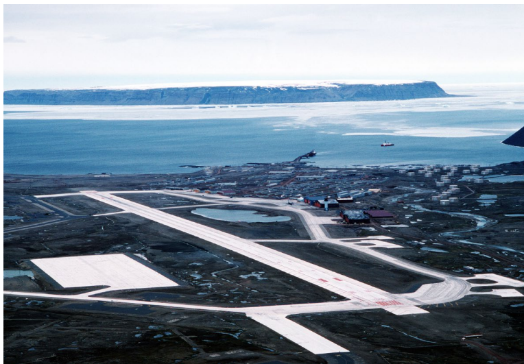
To prevent the thawing of the permafrost underneath the—usually dark asphalt—runway surface, workers painted the entire airfield white to reflect the sun's heat
