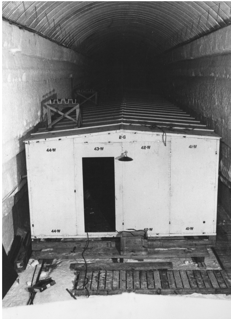
A prefabricated building in one of the tunnels at Camp Century.
