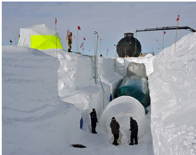
Before covering with snow, balloons are carefully placed and slowly inflated in the open trenches at EastGRIP.
