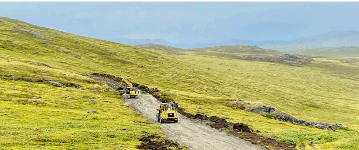
Construction of the road between Kangerlussuaq and Sisimiut, 2020.
