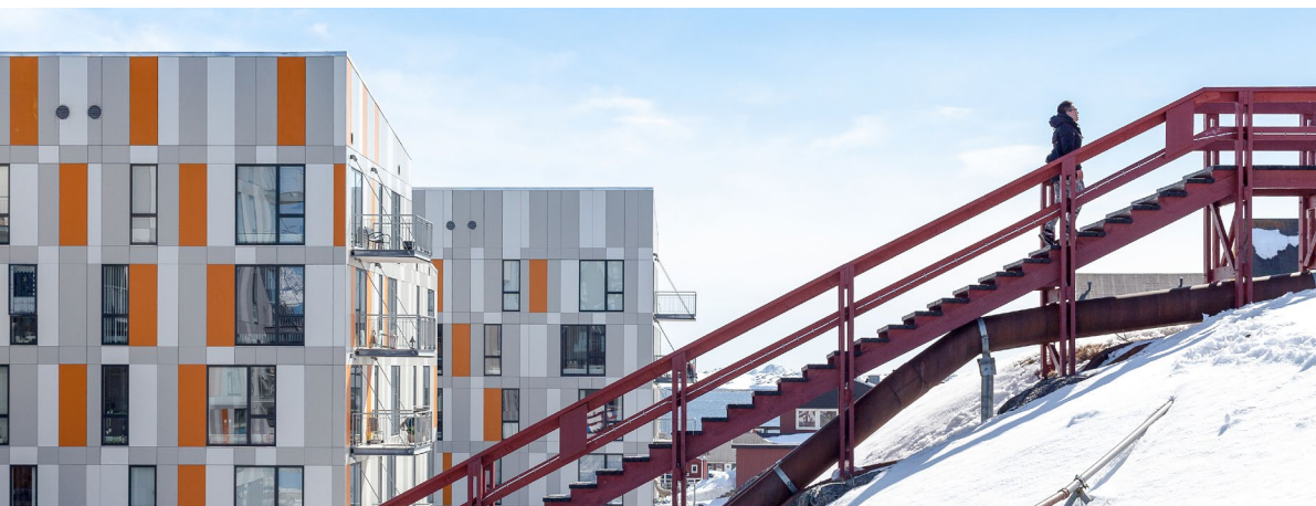
Creative solutions in the urban landscape of Nuuk: a combination of utilities infrastructure and public staircases.
