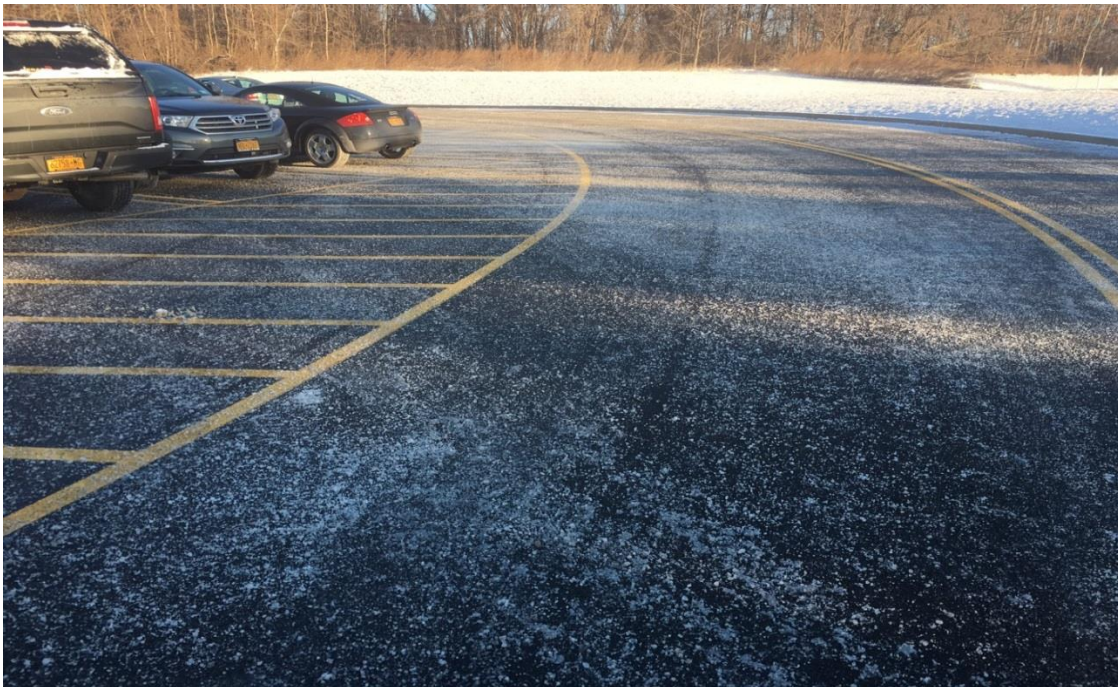
Figure_. Observation of rock salt being over applied in a commercial parking lot.
