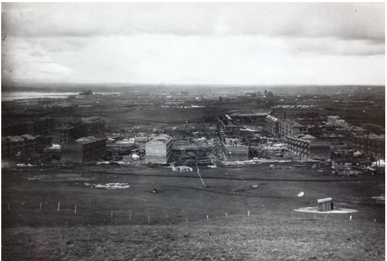
FIGURE 5.51: First buildings of Kirov District under construction with Magnitogorsk factory in background, Gosproekt, 1931-32 Magnitogorskii Kraevedcheskii Muzei
