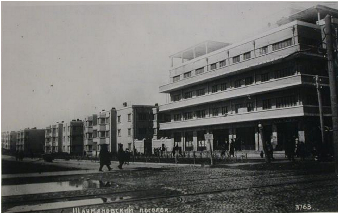
FIGURE 3.38: Armenikend (Shaumian) street view, date unknown Canadian Centre for Architecture, Montreal [PH1998:0011:008]
