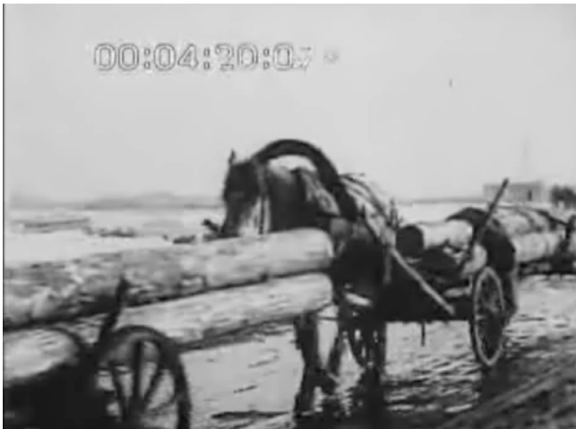
FIGURE 0.2: Horse-drawn building supplies, Kharkiv Tractor Factory site, 1930
