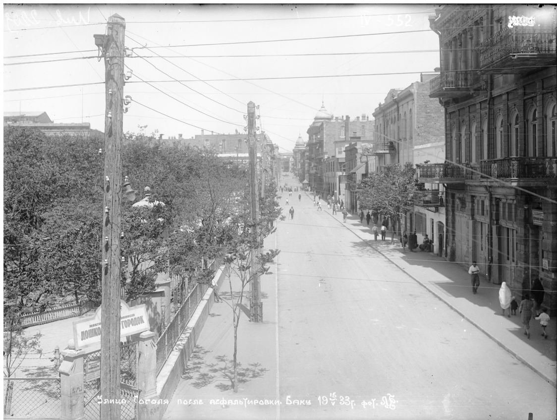
FIGURE 3.16: Gogol Street after reconstruction, May 15, 1933
