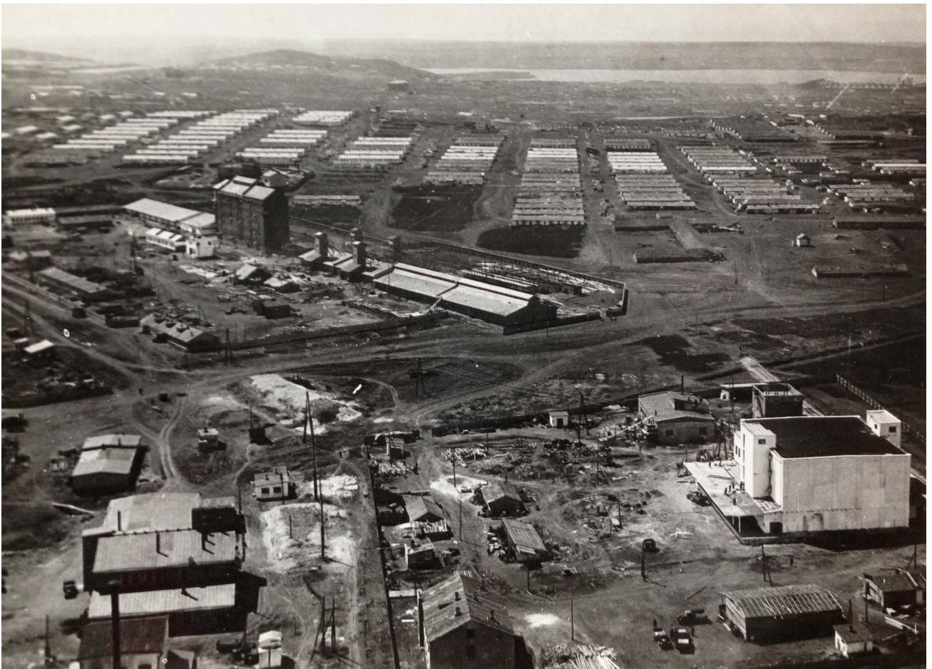
FIGURE 5.40: Aerial view of Magnitogorsk factory construction with rows of wooden barracks in the distance, c. 1930 Magnitogorskii Kraevedcheskii Muzei
