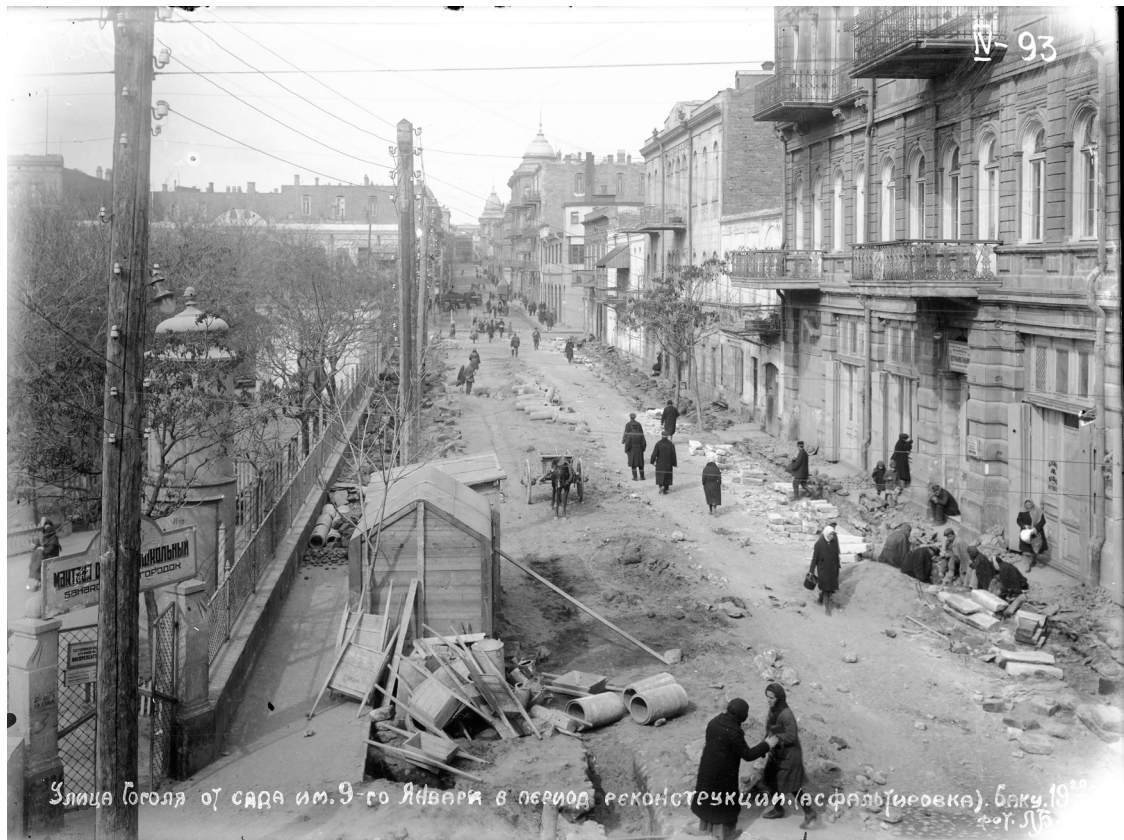
FIGURE 3.15: Gogol Street during reconstruction, February 20, 1933
