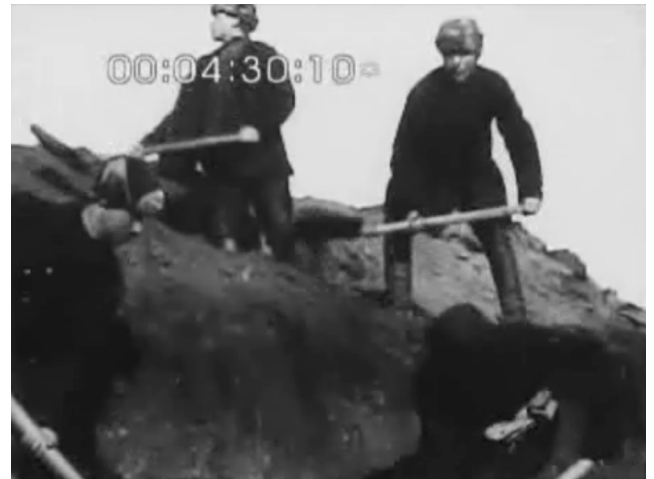
FIGURE 0.3: Foundation pit diggers, Kharkiv Tractor Factory site, 1930
