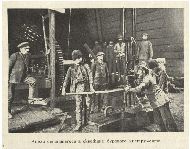
FIGURE 1.10: Catching the borehole remainders with drilling tools
