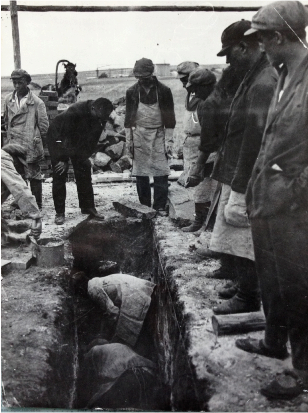
FIGURE 5.39: Laying the first housing foundation, Pionerskaia Street, summer 1930 Magnitogorskii Kraevedcheskii Muzei
