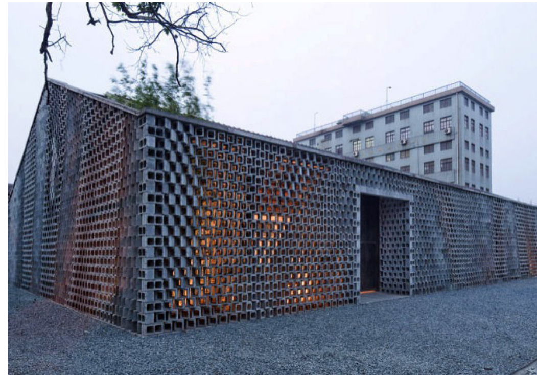
Fig02. Parametric walls used on the renovation of old fabric warehouses in Shanghai. Archi Union Architects. 2010. Image Sheng Zhongha.
