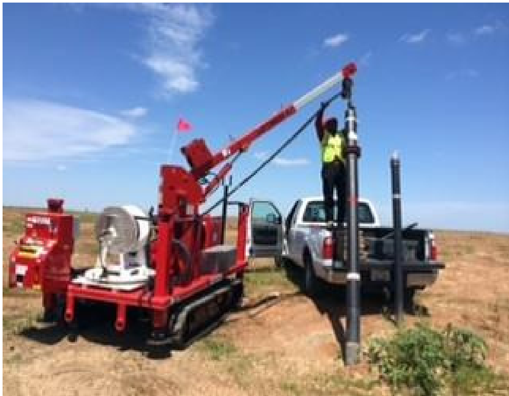
Figure 8. Post-perforation tool being lowered into an extraction well (Stamoulis et al., 2011).
