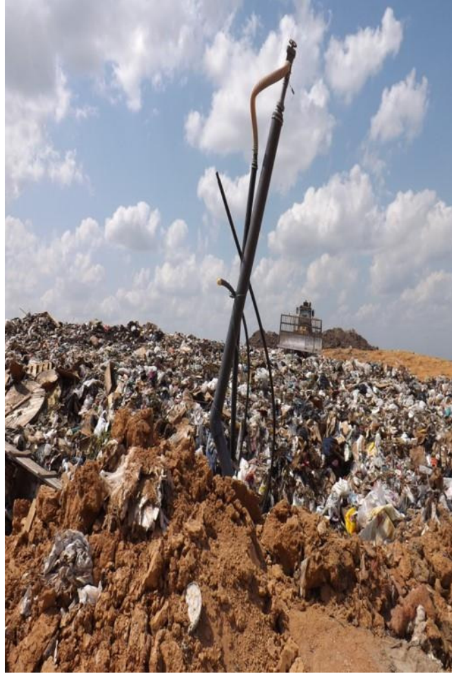
Figure 11. Example of an extended extraction well.
