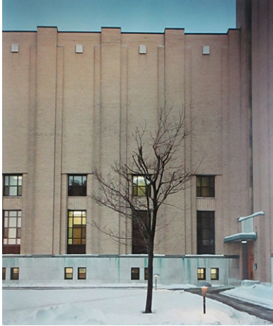
Figure 6.38 A view of the exterior wall of the main pavilion, showing the decorative expression of structure in the cladding of the reinforced concrete piers. Source: Gabor Szilasi, PH1990.0041, Archival Storage II-2 Colour, Collection, CCA.
