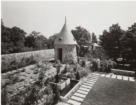
Figure 4.42 Photograph of roof garden with turret containing the stairs leading to the garage. Source: [S. J. Hayward?], ARCH264036, P.6730, folder "P-6730 @ 6751," box P-6669 à 6938, FEC, CCA.
