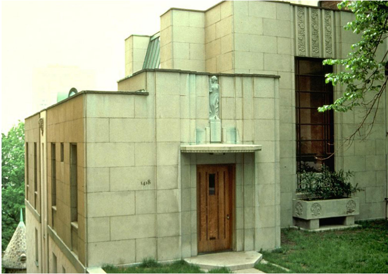
Figure 3.1 A view of the front and the upper part of the side elevations of the Cormier Residence (1930-31) at 1418 Pine Avenue West in Montréal, photographed in 2007. Source: Photography by Denis Robert, “Maison Cormier,” uploaded by Sandra Cohen-Rose and Colin Rose, Flickr Photo Sharing, accessed July 15, 2010, http://www.flickr.com/photos/73416633@N00/1927879504/in/photostream/
