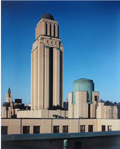
Figure 6.43 A view of the part of the main pavilion's roof line showing the tower and water reservoirs at the tops of staircase towers, photographed 1990. Source: Gabor Szilasi, PH1990.0056_001, Archival Storage II-2 Colour, Collection, CCA.
