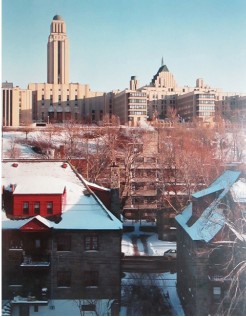
Figure 6.14 A view of the central and west parts of the main pavilion, overlooking the residential neighborhood situated lower on the slope of Mount Royal, c.1990.
