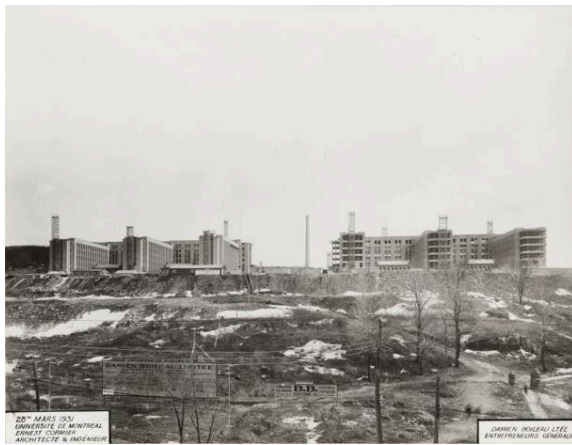
Figure 1.6 A photo of the construction site of the Université de Montréal, taken on March 28, 1931, showing the incomplete state of the pavilion, particularly its central zone. The chimney in the center is that of the temporary powerhouse at the rear of the site. Source: S. J. Hayward Photographic Studios, ARCH264436, P.1874, box Cormier 01-2402-01P-#2402, FEC, CCA.
