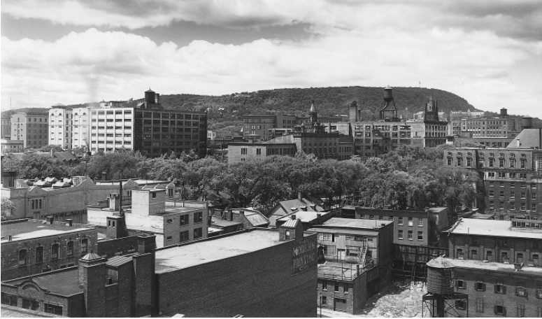
Figure 6.42 Photograph of Montréal looking north from the Southam Press Building, 1926-27, showing the large water reservoirs that were a standard feature on the roofs of large buildings at the time. Source: Wm. Notman & Son, VIEW-24047 © McCord Museum.
