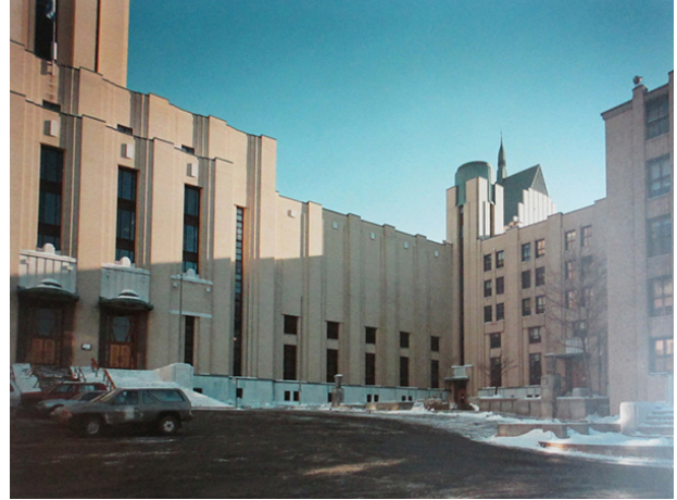
Figure 6.39 A view of the western corner of the central courtyard of the UdeM, showing the decorative treatment given to the piers through the handling of the brickwork. Source: Gabor Szilasi, PH1990.0042, Archival Storage II-2 Colour, Collection, CCA.
