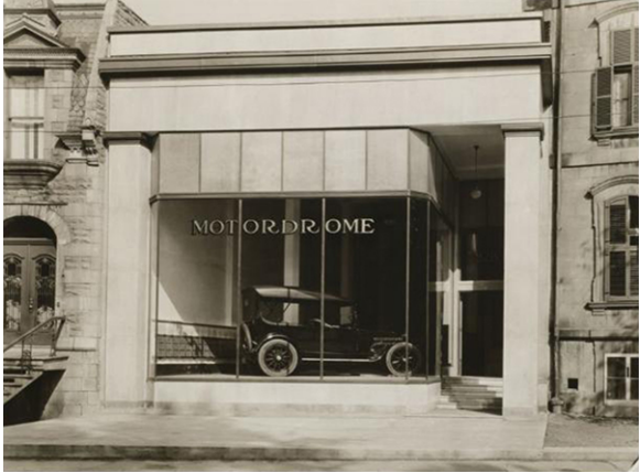
Figure 3.22 A photograph of the front facade of the Motordrome (the Montée du Zouave Garage) on Sherbrooke Street in Montréal, by Ernest Cormier (1919-20), taken c.1920. Source: S. J. Hayward Studios, ARCH252070, Cormier SNP 3, EC 089, box 01-Photos-03P, FEC, CCA.
