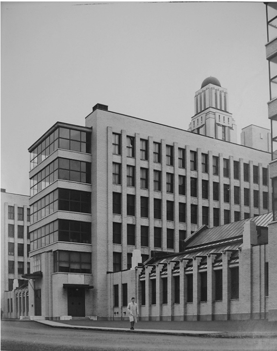
Figure 6.37 A photograph wing B of the hospital connected to adjacent wings through the low single-story connectors intended to house the outpatient clinics, (undated).
