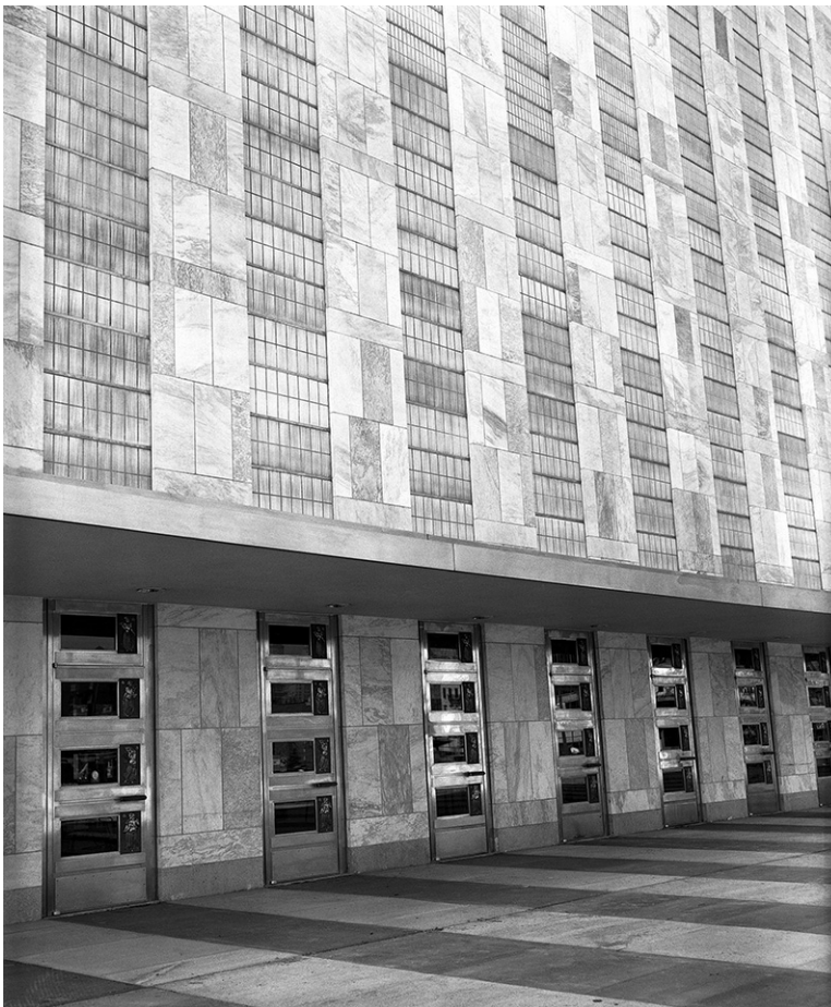
Figure 7.5 Photograph of the main public entrance to the General Assembly Building, showing the seven nickel-bronze doors designed by Cormier and the glass and marble wall of the north facade, photographed in 1962. Source: UN Photo/MB, Photo #336365, October 1, 1962.
