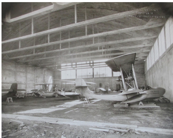
Figure 3.26 A photograph of the interior of the reinforced concrete seaplane hangar (1928-30), that Cormier designed for the Compagnie Aérienne Franco-Canadienne, (undated). Source: [Unknown photographer], ARCH258693, folder 906/A-25, box 001-2011-037 T, FEC, CCA.
