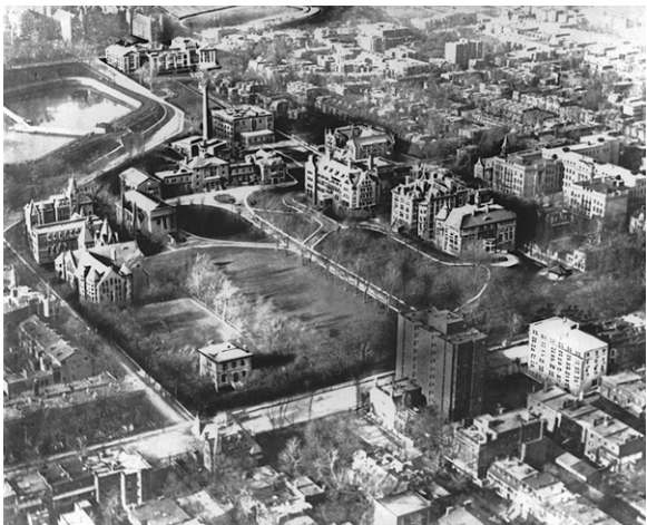
Figure 5.13 Aerial view of the campus of McGill University, Montréal, QC, 1921. Source: Anonymous, photograph, 1921, MP-0000.1877.2 © McCord Museum.
