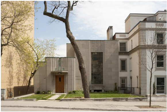
Figure 4.8 Photograph of the Pine Avenue West elevation of the Cormier Residence showing it mitoyen to the Gillespie house, photographed in 2012.
