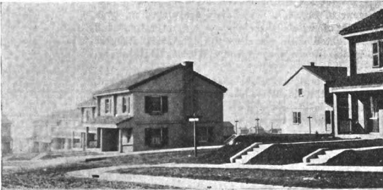
Fig. 76. Plates from "281 Fireproof Dwellings Built of Large Precast Concrete Units", showing a photograph of the first pair of row-houses completed at Youngstown, prior to the addition of mass produced building components, such as windows and gutters (top) and photograph of a group of row-house units, after the mass produced components were added (bottom). Compare to Figs. 149 and 167. Source: "281 Fireproof Dwellings Built of Large Precast Concrete Units." Concrete 14, no. 1 (1919): 3-8.
