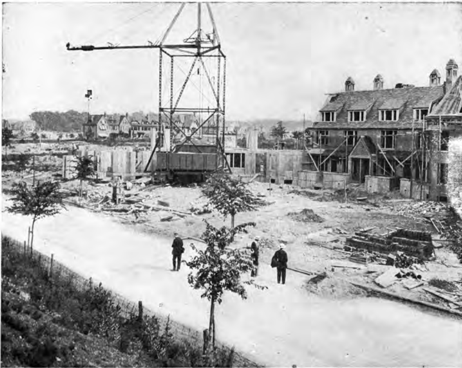
Taking Wall Blocks from Transfer Car. Group II, Forest Hills Gardens.
