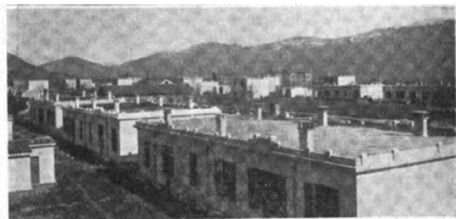
Fig. 64. Plates from Small, "Poured Houses in Holland", showing the unit developed through collaboration between Harms, Small, Hanna and Berlage (left) and plates from Harms, "Building Concrete Industrial Houses by Harms System in France", showing the applied ornamentation on the units in France. Source: Small, George E. "Poured Houses in Holland." Cement Age - Concrete Engineering XIV, no. 2 (February, 1912): 63-67; Harms, Henry J. "Building Concrete Industrial Houses by Harms-System: Second Article Describes Layout of Work, Equipment and Methods Used." Concrete 12, no. 2 (February, 1918): 41-46.
