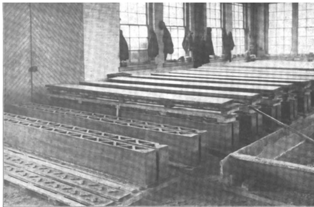
Fig. 80.—Molding of Visintini Girders. (See p. 155.)
