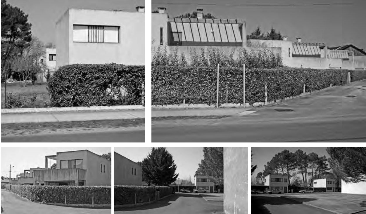
Fig. 110. Photographic study of the experience of the houses in series at Lege, 2012. Source: Author.
