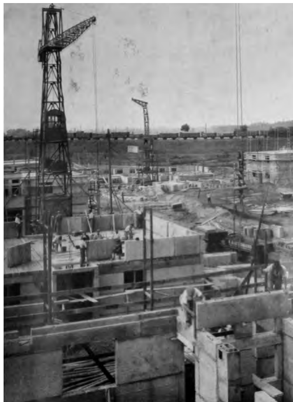
Fig. 204. Plate from Das Neue Frankfurt showing assembly of panels at Mammolsheinerstrasse, 1928. Source: Das Neue Frankfurt 8 (August 1928). 122.
