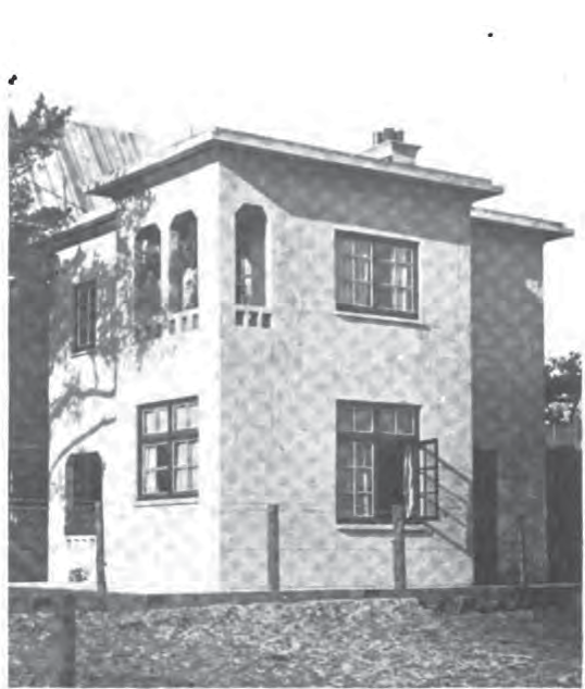
FIG. 1—THE COMPLETED HOUSE AT SANT-POORT, HOLLAND. The concrete for this house was placed in one continuous six-hour pouring.
