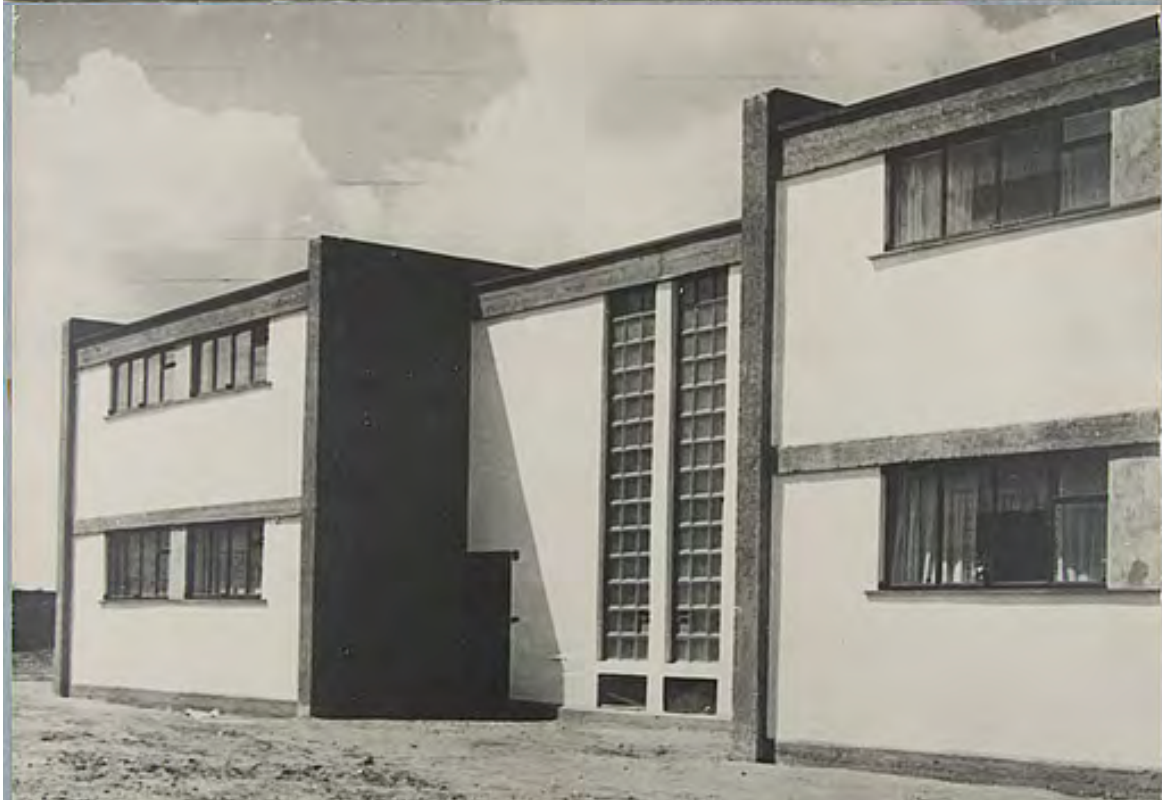
Fig. 158. Walter Gropius. Photograph of a series of Type II's, under construction, with the new three hundred and sixty centimeter module clearly visible (top) and photograph of a pair of Type II's, with finishes, showing the expression of load-bearing structure (bottom), 1927-28. Sources: HAM/B-RM BRGA.22.85; HAM/B-RM BRGA.22.33.
