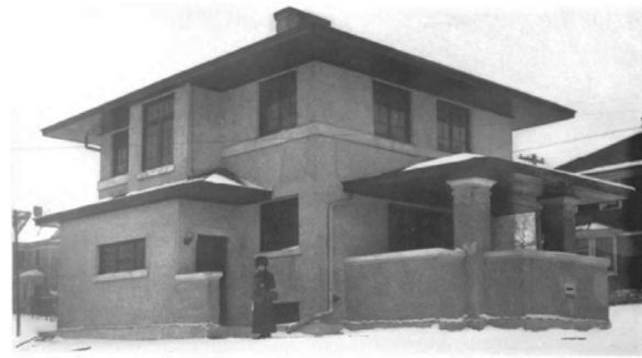
Residence of G. L. Calkins, Oklawaha, Fla. Harry E. Thross, Architect House constructed with Van Gulder hollow concrete walls. Mixture and plaster applied directly to walls.
