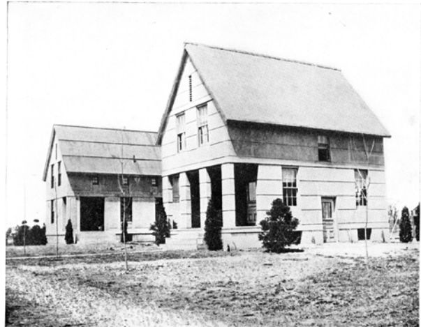
Houses at Seawarren, N. J. Erected 1908-9. Standardized Hollow Concrete Construction Throughout.
