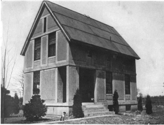
Workers' College, Sewaren, N. J. Starr Foundation Homes Co. Greene A. Barber, Architect, N. Y. A fireproof, sanitary, and indestructible house, built throughout of huge, precast concrete slabs, and intended to solve the problem of better living conditions for working classes at minimum cost.
