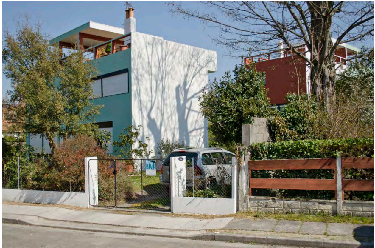
Fig. 127. Le Corbusier. Perspectival study of position of unit and pedestrian path on parcel 14, looking west (top) and photograph of recently renovated unit on parcel 14, looking east (bottom). Sources: FLC 19859; Author, 2012.
