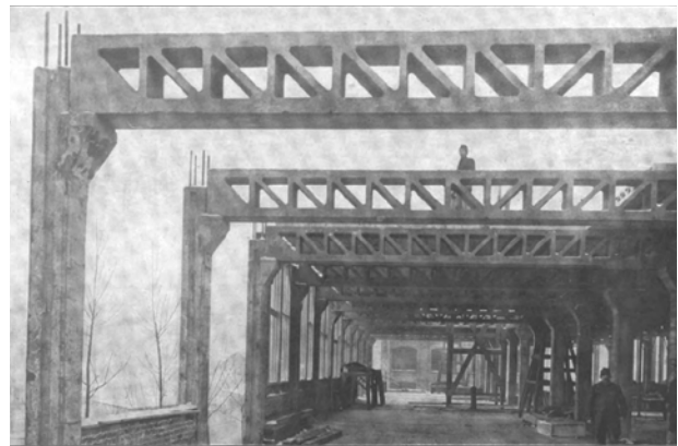
Fig. 77.—View of Visintini Columns and Girders in Textile Machine Shop. (See p. 121.)
