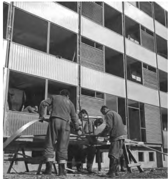
Fig. 236. The JU 61 aluminum "membrane" (left) and the assembly of the JU 61 façade (right), 1963. Source: Private Archive, Bogdan Budimirov.
