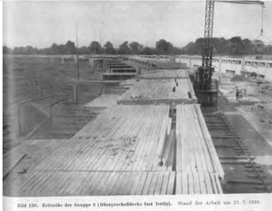
Fig. 172. W. Gropius. Progress photos showing deck for ground floor being installed, July 19 and July 21, 1928, upper floor walls being erected, July 23, 1928 and roof deck being installed July 31, 1928 as well as two progress charts, used by the contractor (right), used to manage and record the construction of Group 8 Type IV. Source: "Bericht Über Die Versuchssiedlung in Dessau." RFG Sonderheft Nr. 7, no. Gruppe IV NR. 4 (April 1929).
