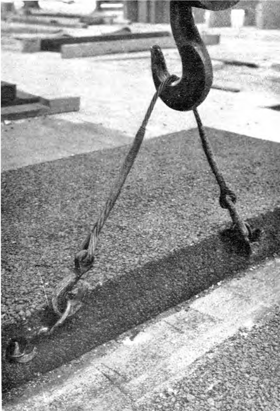
Fig. 192. Plate from RFG report showing typical one-meter wide panel, with rough finish and reinforcing, for transport, visible.
