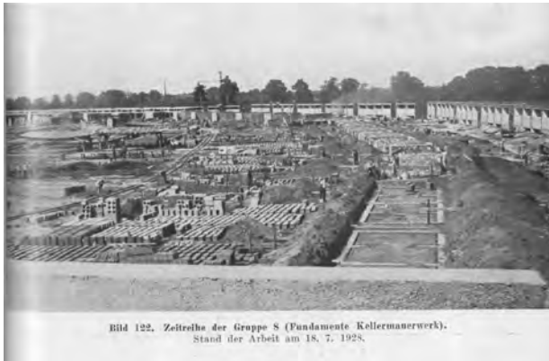
Fig. 171. W. Gropius. Progress photos showing the cellar ceiling being installed, July 14, 1928, first level masonry walls being constructed, July 15 and July 16, 1928, foundation of cellar (missdated, out of sequence) as well as a progress chart, used by the contractor (right), used to manage and record the construction of Group 8 Type IV. Source: "Bericht Über Die Versuchssiedlung in Dessau." RFG Sonderheft Nr. 7, no. Gruppe IV NR. 4 (April 1929).
