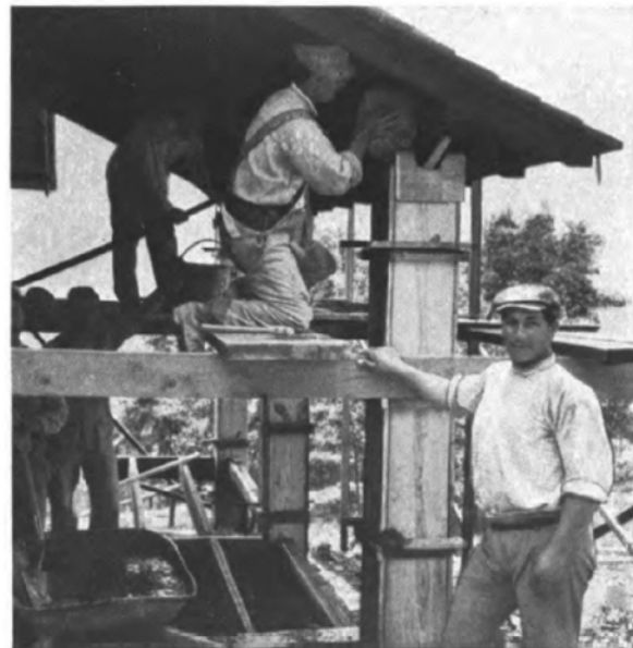
Pouring concrete into a column form. [ 78 ]
