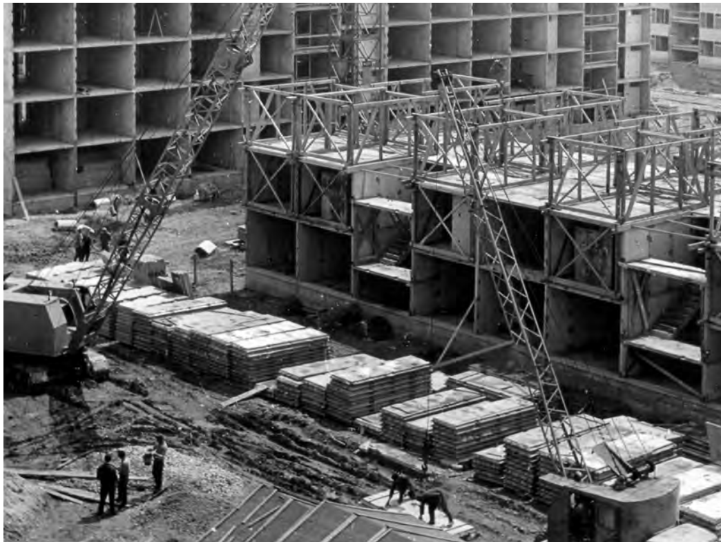
Fig. 241. Drawing showing locations of JU 61 panels in their delivered and assembled positions, 1961 (top) and photograph of the application of this projection system at Borongaj Settlement, Zagreb, later 1962 (bottom).
