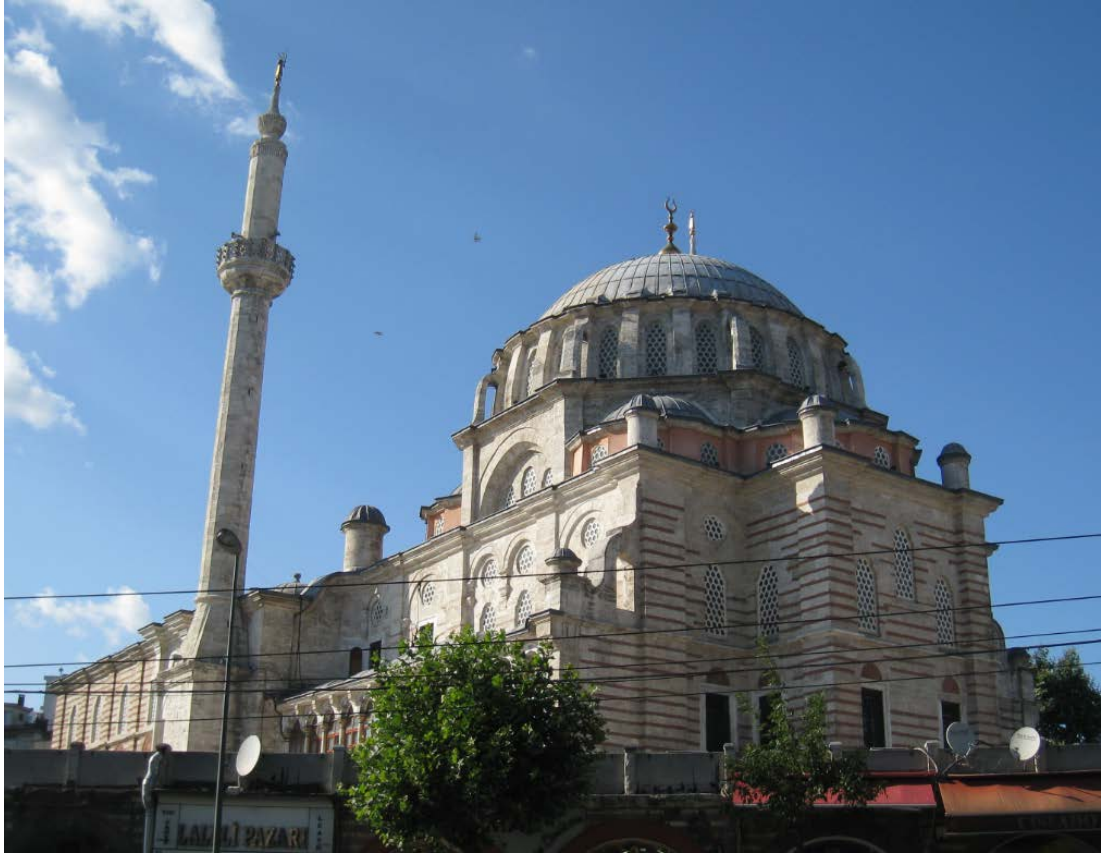
Figure 269. Laleli Mosque, from the south.
