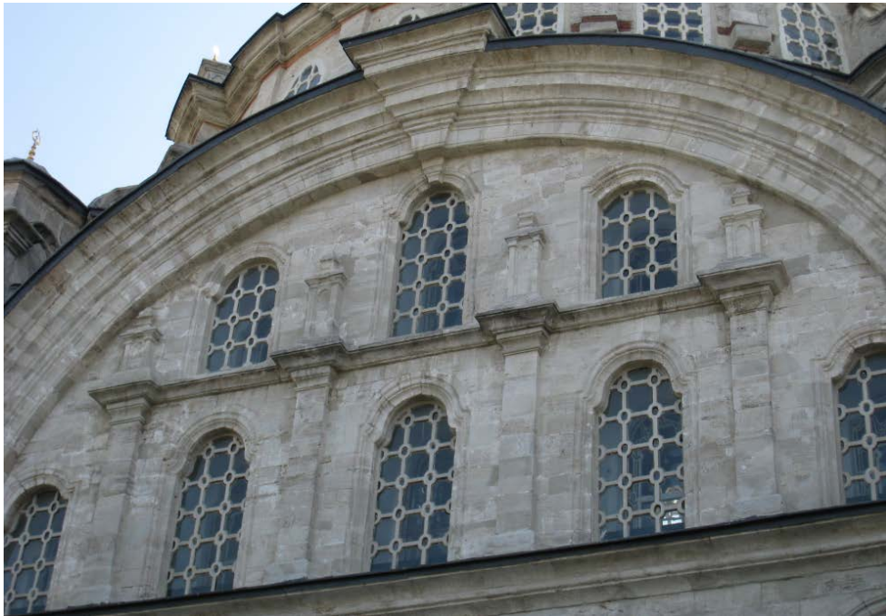
Figure 454. Selimiye Mosque, baldachin tympanum.
