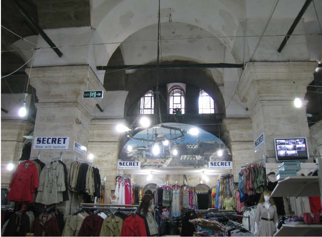
Figure 277. Laleli Complex, vaulted basement.
