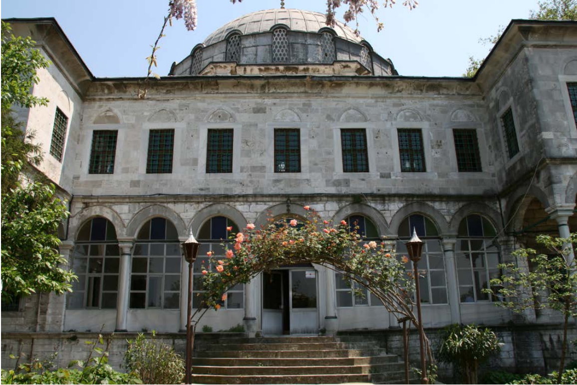
Figure 404. Beylerbeyi Mosque, pavilion façade.
