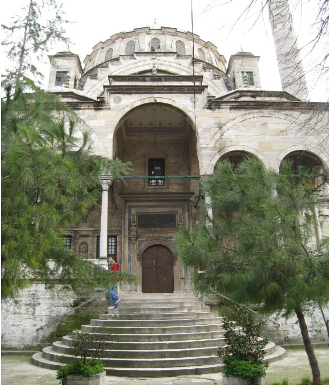
Figure 239. Ayazma Mosque, entrance portico and stairway.
