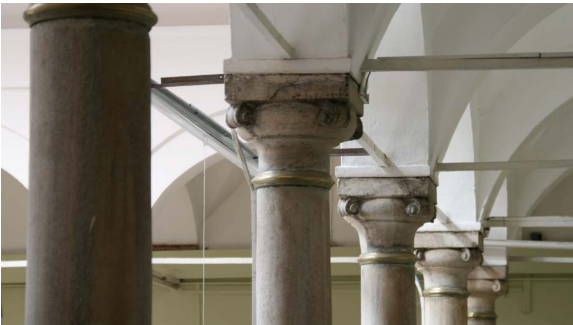
Figure 379. Hamidiye Complex, columns of the madrasa.
