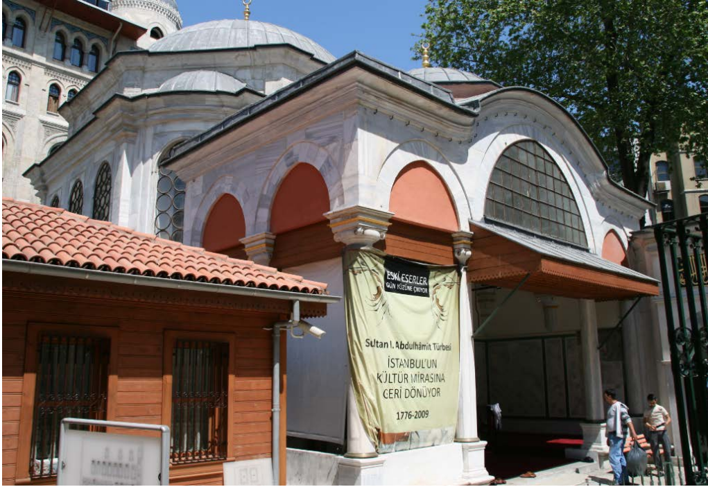
Figure 387. Hamidiye Complex, tomb, exterior looking towards the entrance portico.
