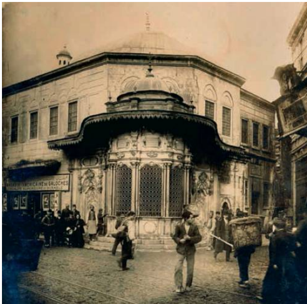
Figure 366. Hamidiye Complex, late 19th–early 20th-century photograph of the sebil and primary school in their original form, with 19th-century rusticated cladding on the walls. From Bülbül, “Hamidiye İmaretı,” 12.
