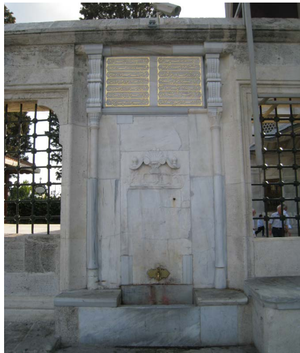
Figure 59. Inauthentic modern restoration of the fountain of Nişancı Ahmed Pasha, southwest wall of the Fatih Complex cemetery, Istanbul.
