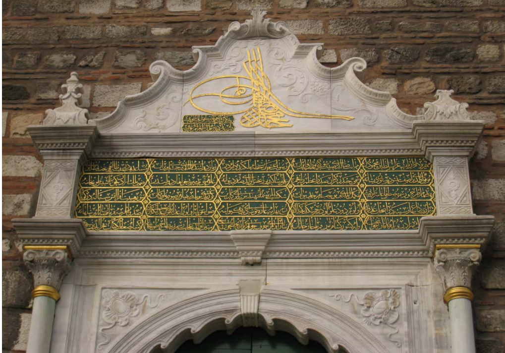
Figure 84. Tophane, upper part of the entrance.
