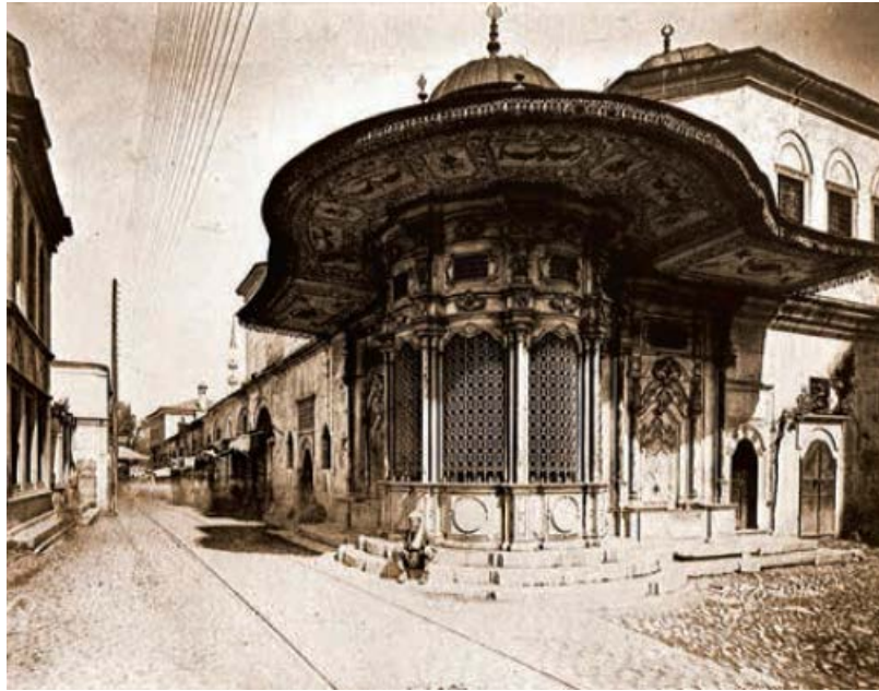
Figure 365. Hamidiye Complex, late 19th–early 20th century photograph of the sebil, primary school, and imaret in their original form,. From Bülbül, “Hamidiye İmaretı,” 12.
