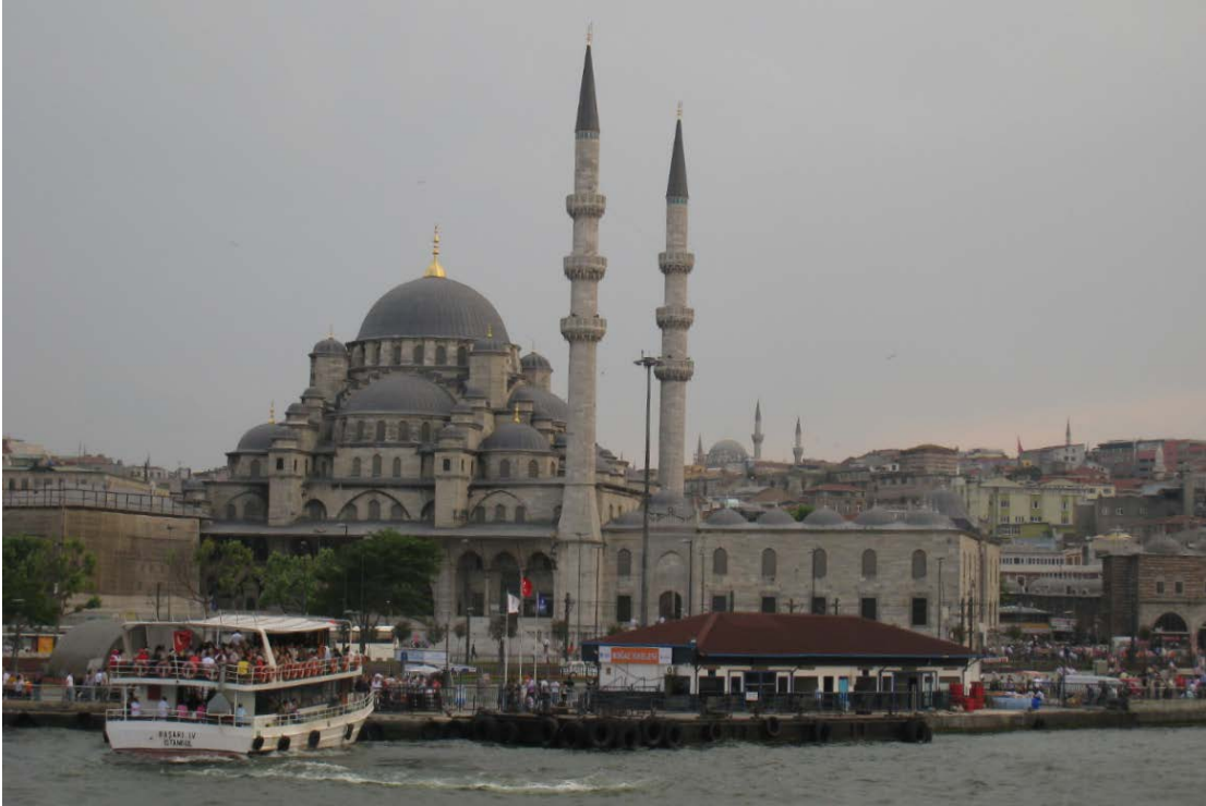
Figure 134. Yeni Cami (architects: Davud Agha and Dalgıç Ahmed Agha), Eminönü, Istanbul, 1597–1665.
