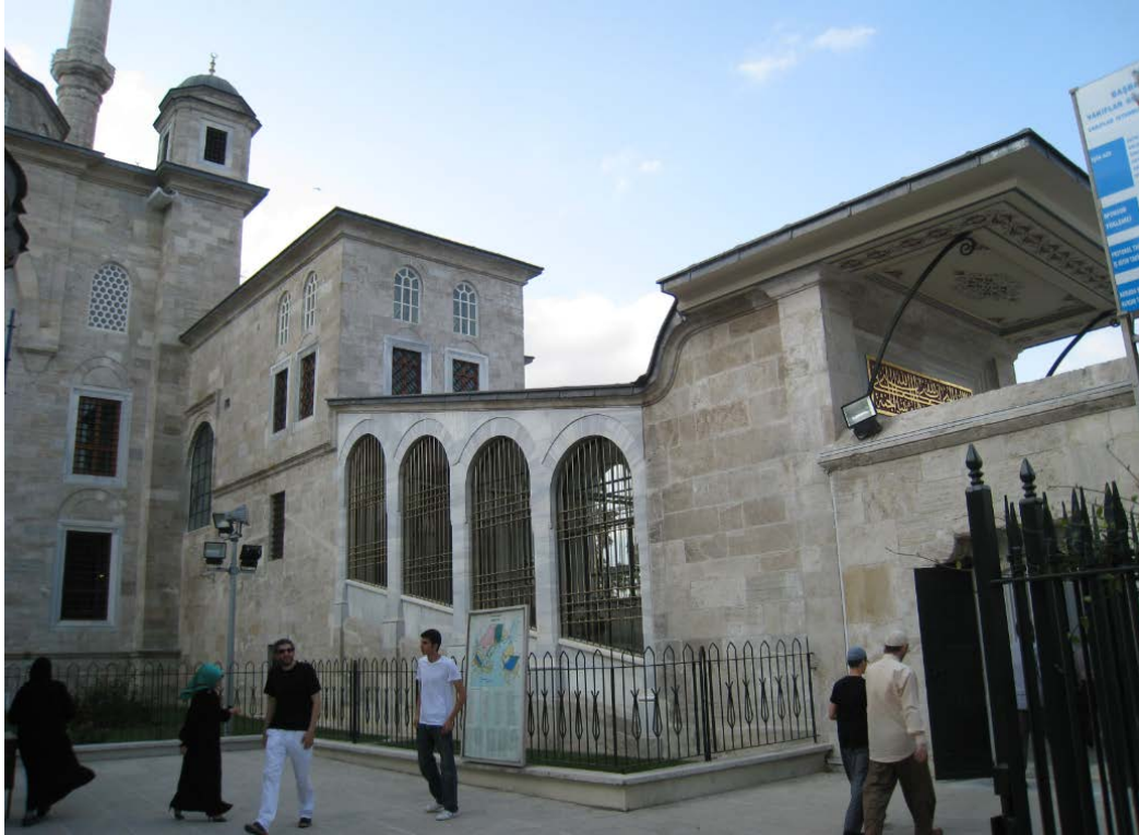
Figure 342. Fatih Mosque, sultan's pavilion, ramp.
