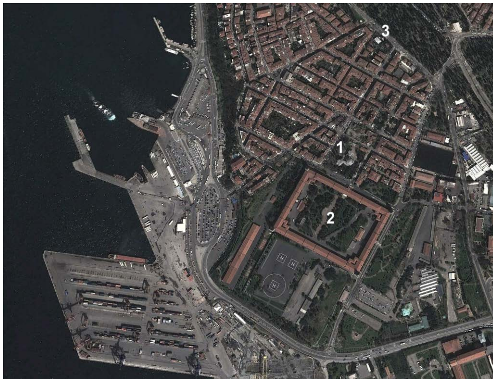
Figure 450. Aerial view of the Selimiye Mosque and its environs: 1. mosque; 2. Nakşibendi lodge (now the Küçük Selimiye Çiçekçi Mosque); 3. barracks. From Google Earth.
